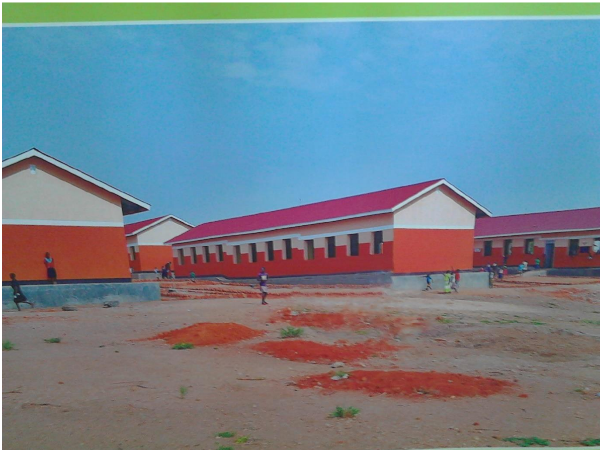
Figure 8: Classroom Blocks Constructed by Finn Church Aid (FCA)
