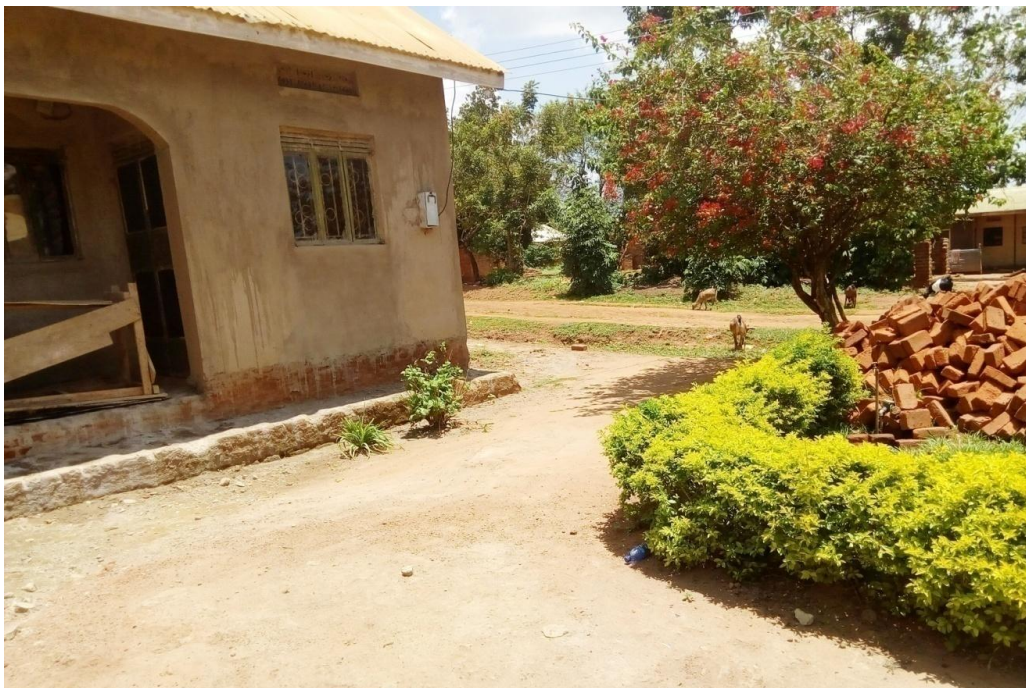
Figure 4.7 shows house construction and electricity installed in home stead for sugarcane grower in Wakalenge village.
