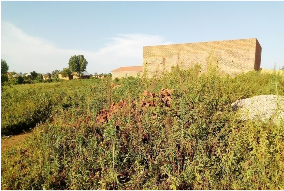
Figure 4.6 shows a house for sugarcane grower under construction in Nakabango village
