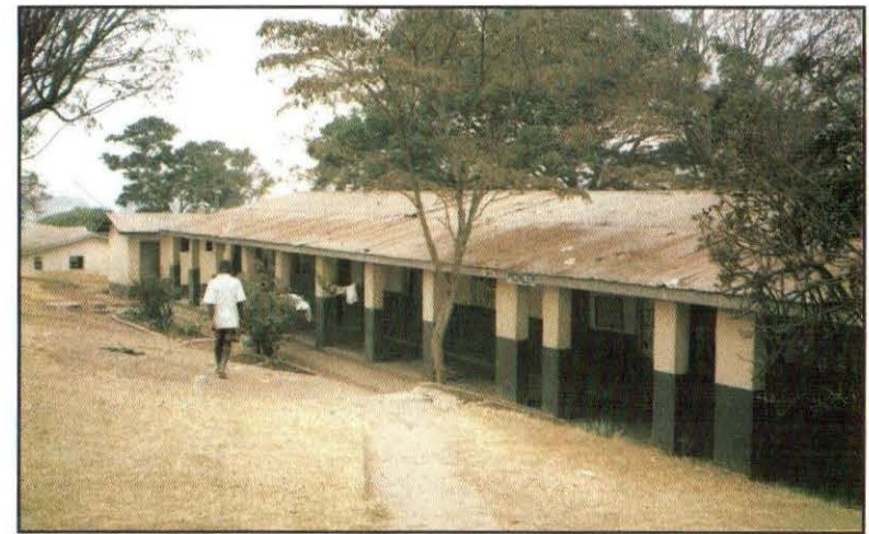
One of the two Hostels built for the GTTC at Ntare School in Mbarara. Photo courtesy D. K. Mulindwa
