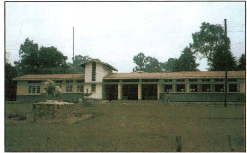
The renovated GTTC Assembly Hall at Ntare School in Mbarara Photo courtesy D. K. Mulindwa
