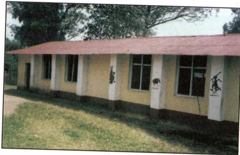
The renovated block that housed the GTTC at Nyakasura School Photo courtesy C. B. Adupa
