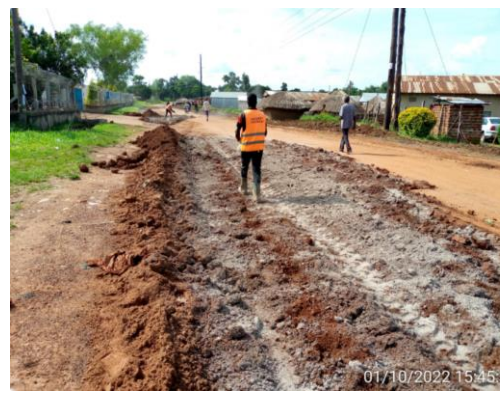
Figure 2. 7: Lime application by casual labourers.
