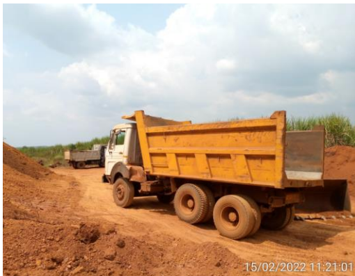
Figure A. 3: TATA 2516C at the quarry site.
