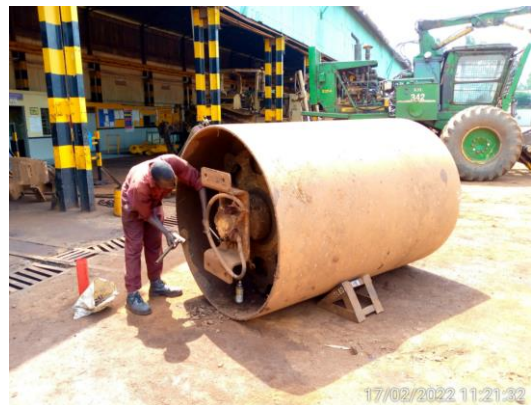
Figure A. 12: Repair of the Ingersoll rand vibrator drum.
