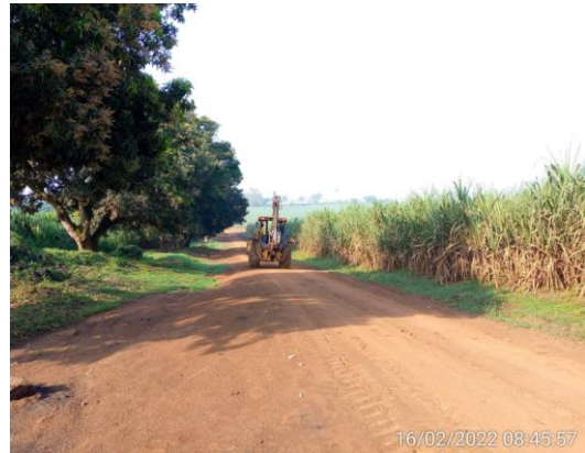
Figure A. 8: The JCB 3CX heading out to site.
