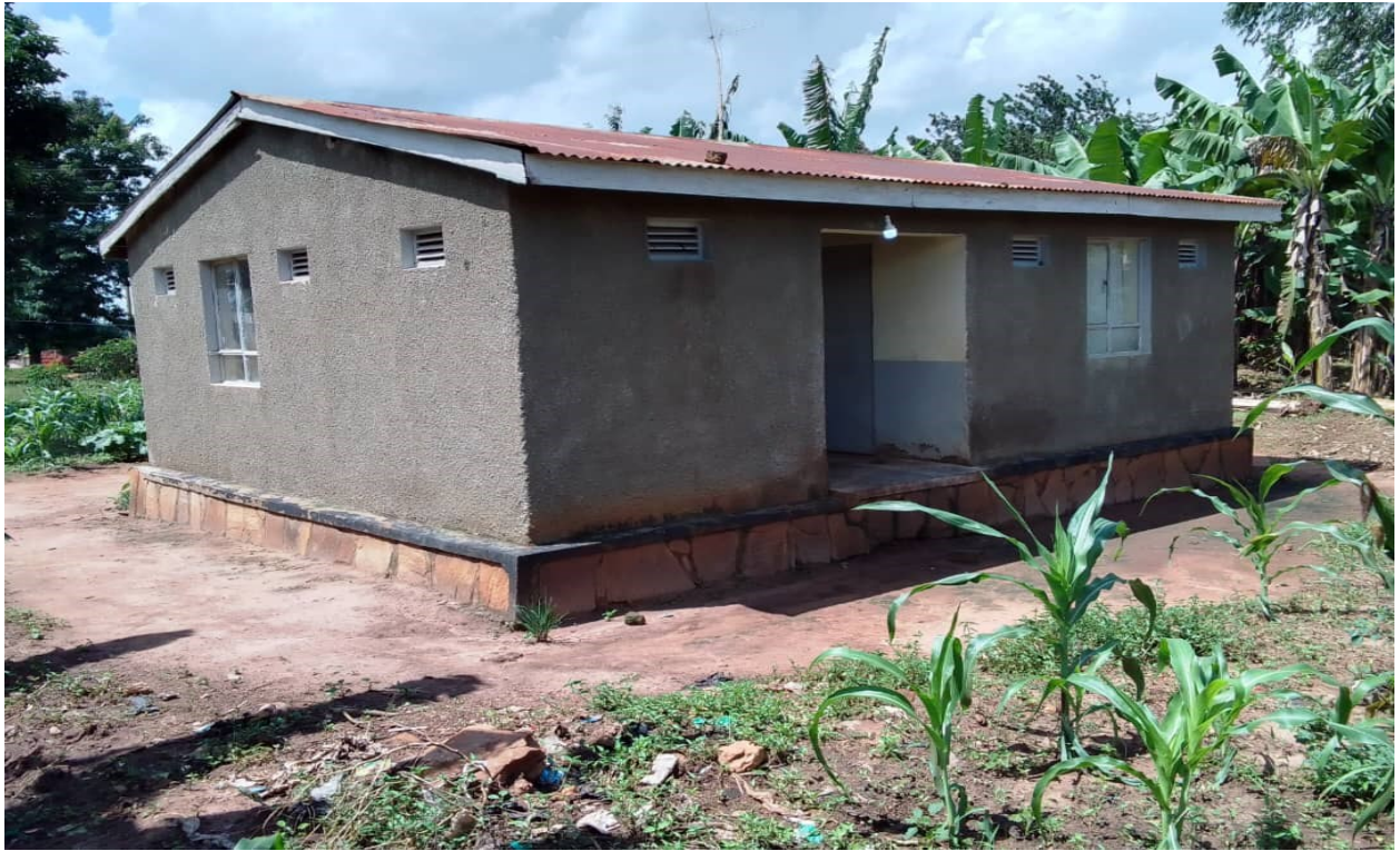
Figure 4.3: An example of a house construction and solar Panel installed in a home stead for a sugarcane grower in Kisasi village
