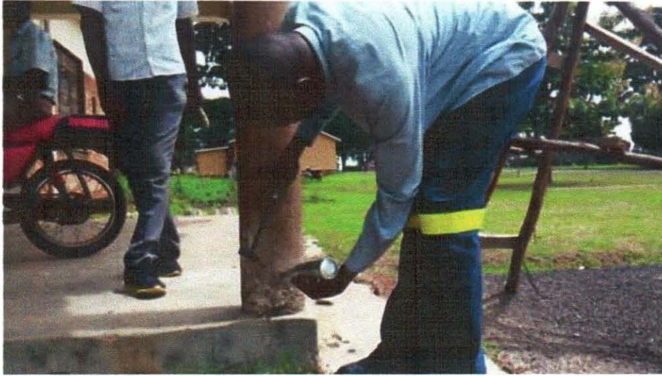
Figure 7.3: Cracks at the bottom of the Column at the District Health Drug Store.
