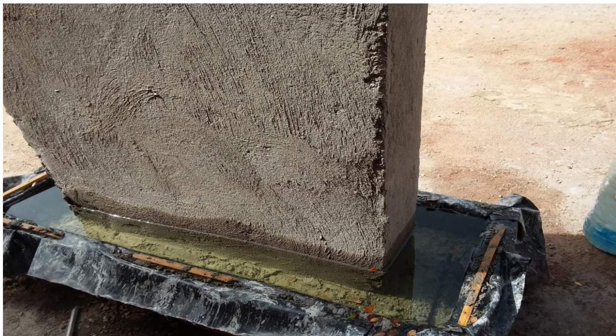
Figure A3.5: showing moisture rise through the researcher's experimental model 1, simulating a masonry wall, at Kyambogo University Soil Laboratory.
