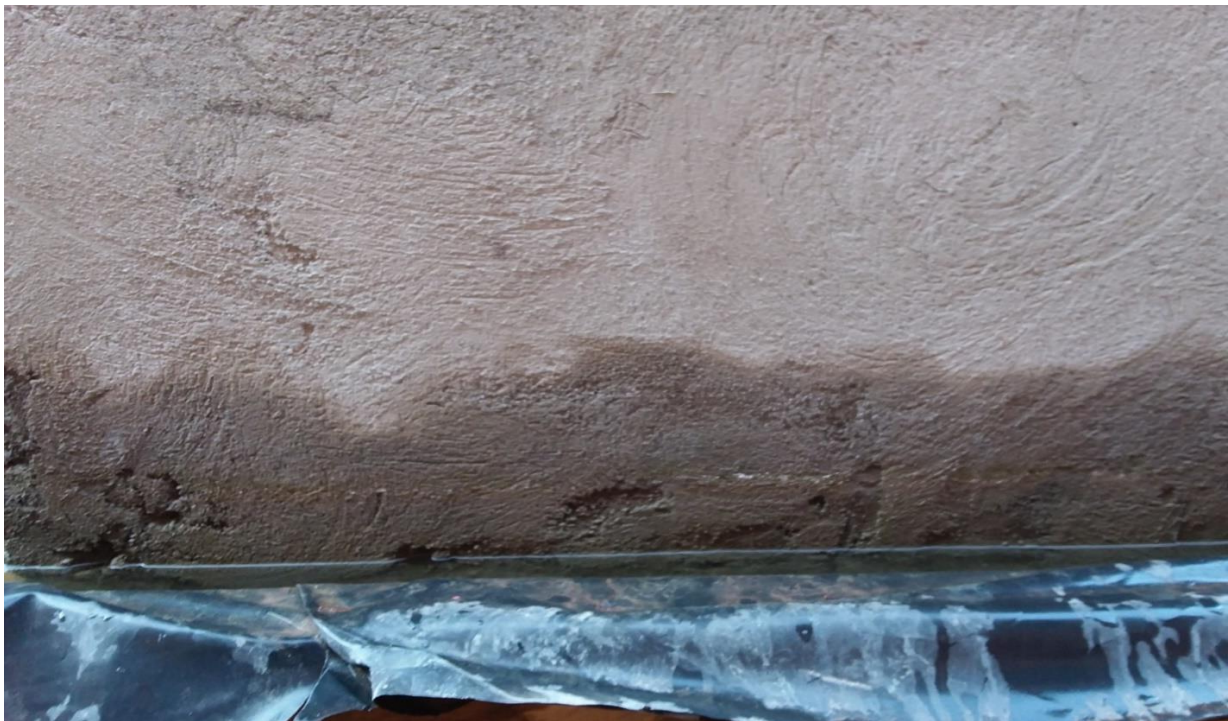
Figure A3.8: showing moisture rise through the researcher's experimental model R simulating a masonry wall, at Kyambogo University Soil Laboratory
