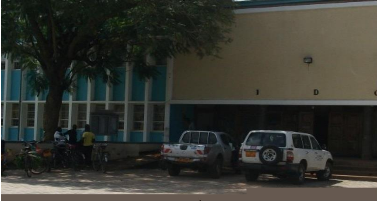
Figure 1.2: Photo of Lira District Local Government Headquarters built in the 60's, & 70's showing no wall defects
