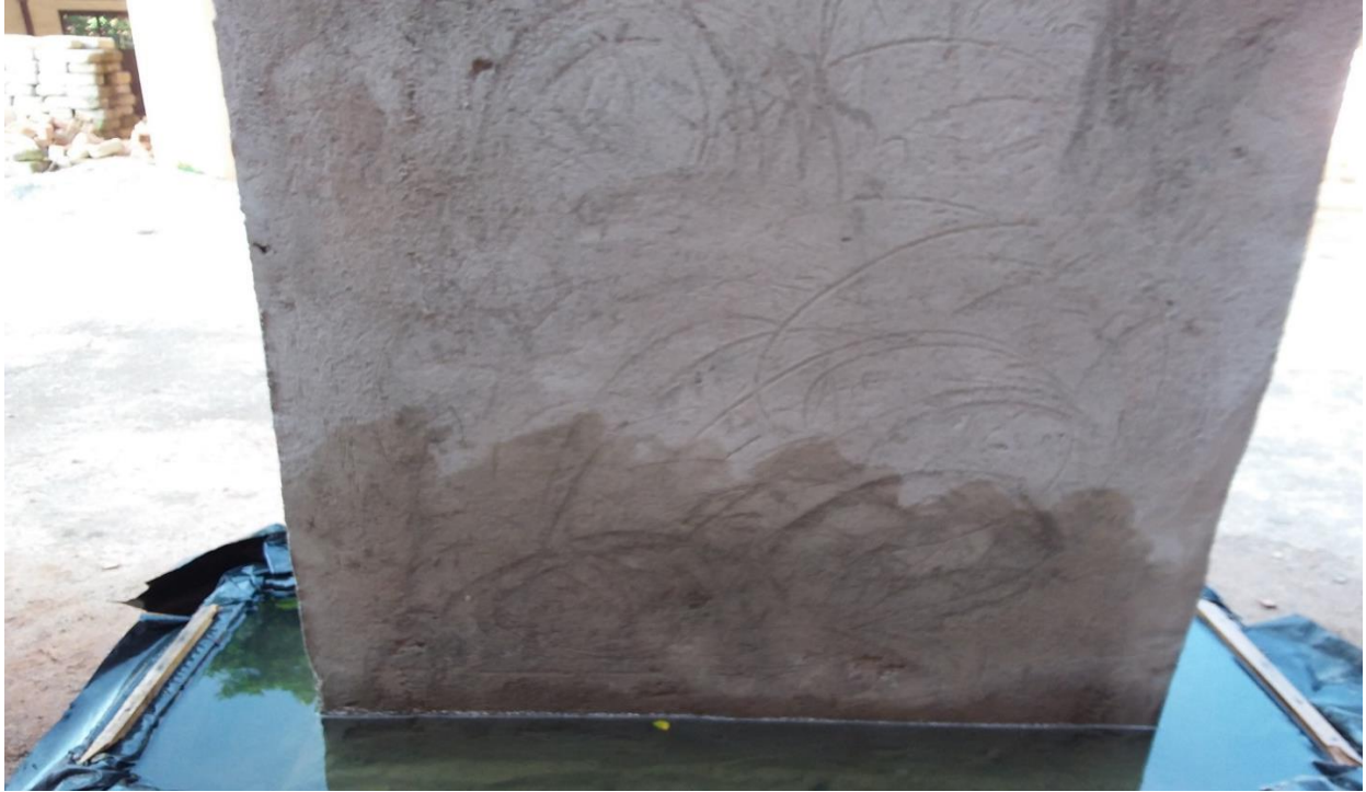
Figure A3.7: showing moisture rise through the researcher's experimental model 4 simulating a masonry wall, at Kyambogo University Soil Laboratory
