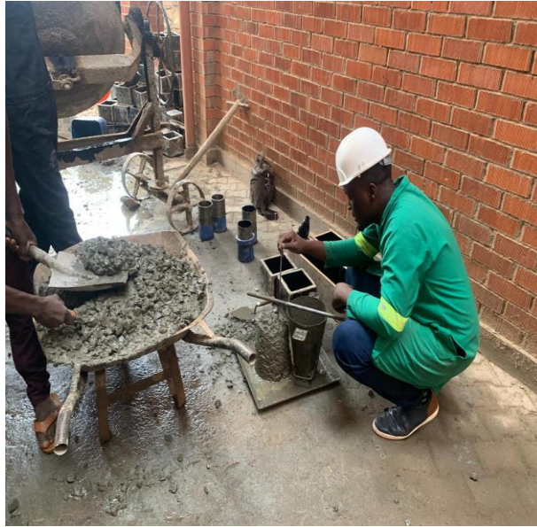
Figure 3.6 Slump test after concrete mixing
