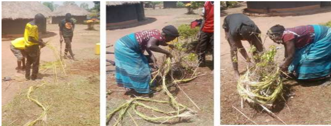
Figure 4.27: Woven spear grass (obiya) was prepared for binding Okango. Sources: Researcher (Pukony sub-county)
