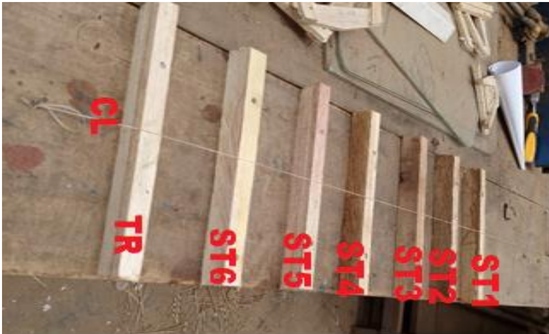
A building jig prepared to receive frames Source: Primary Data 2022
