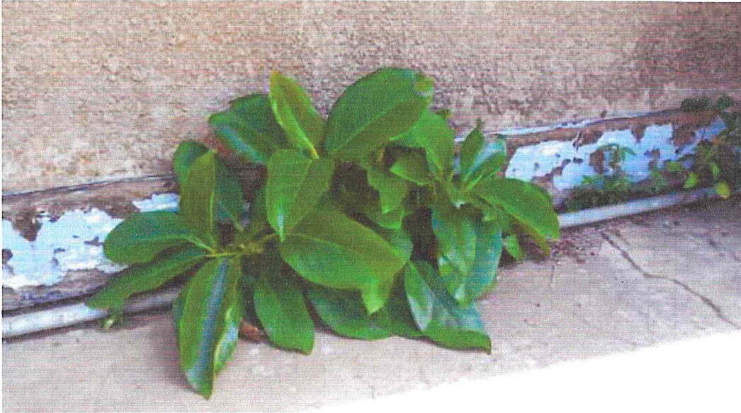
Figure 7.5: Plant growth at the External wall of the Operating Theatre at Amuria H/C IV.
