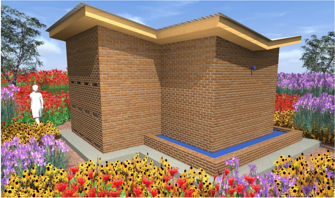
Figure 4.8.48 Water trough around the water tank that will be used during dry seasons.
