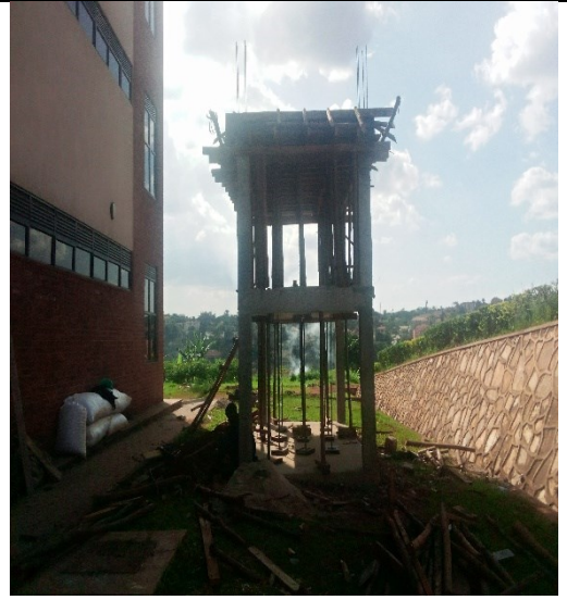
Experiment model before casting upper slab
