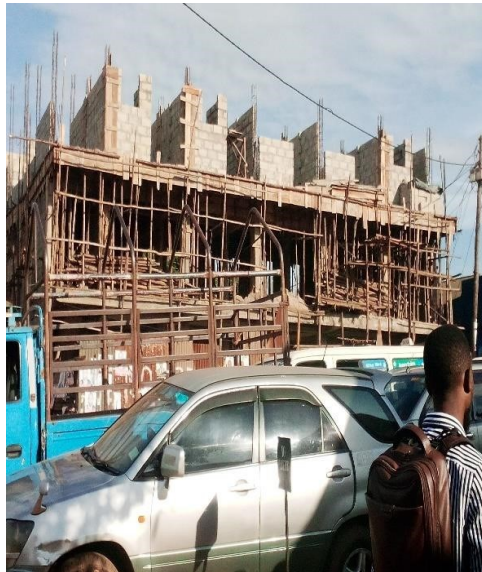
Construction loads; props and slab
