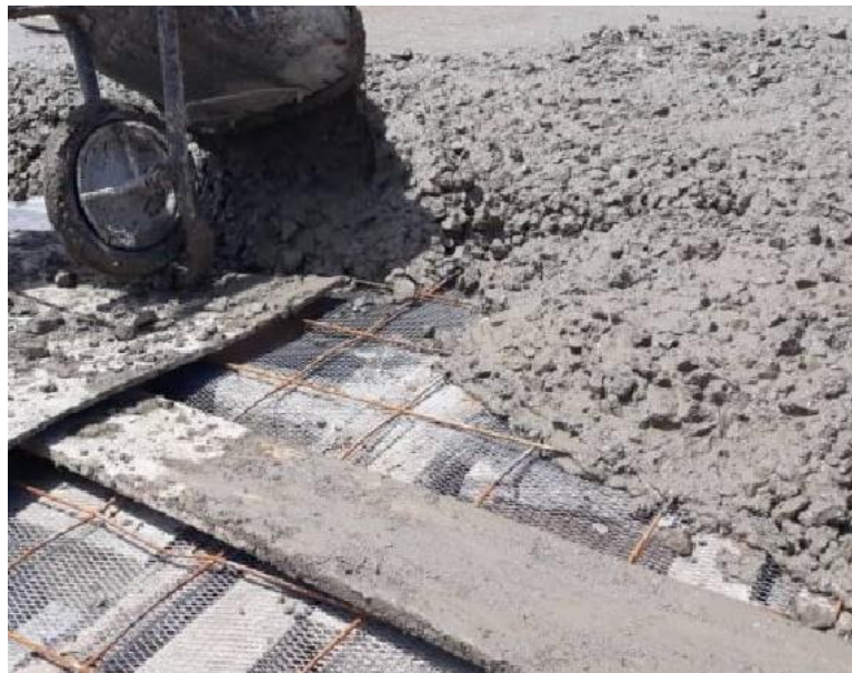
Figure 1.4: Casting the hybrid slab concrete topping.
