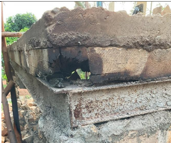
Figure 4.13: The concrete returning to normal with no observed curling
