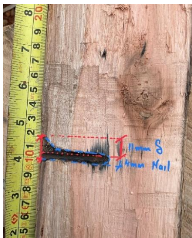
Figure 4.38 Timber concrete dowel connection timber failure
