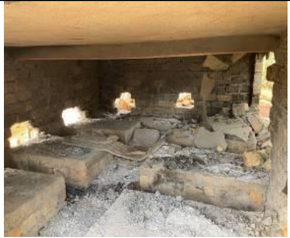
Figure 4.10: Deflection in the central I-Beam
