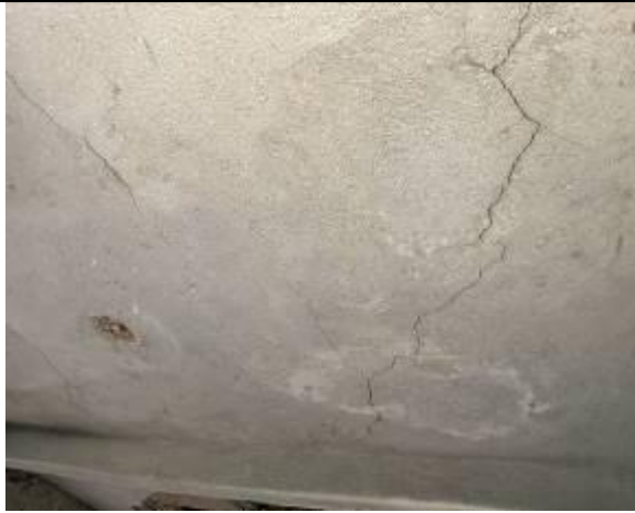
Figure 4.9: Plaster spalling
