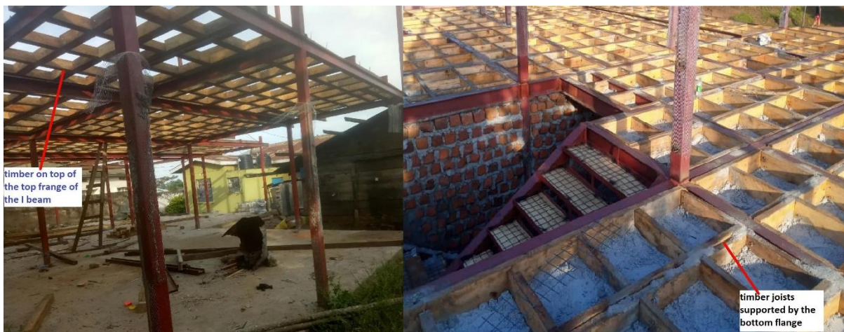
Figure 1.3: Support conditions for timber frame.
