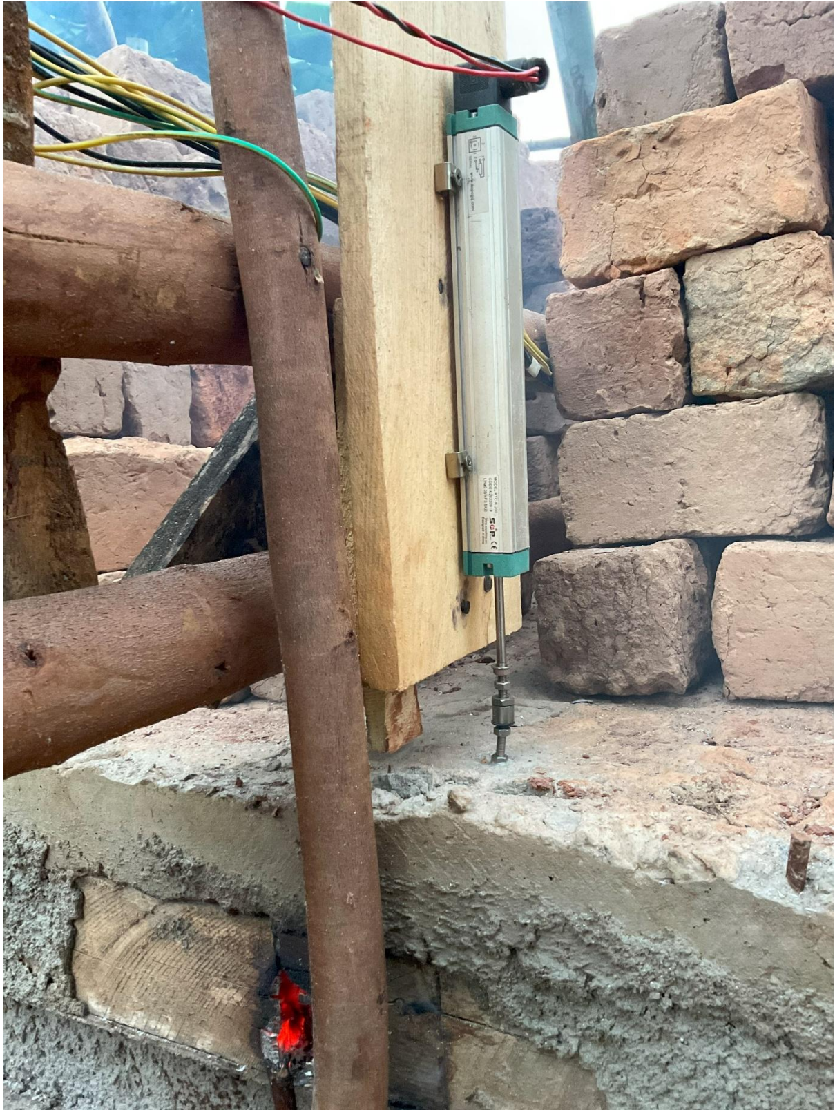
Figure D.4: Linear variable displacement transformer (LVDT) mounted on the slab to measure deformation
