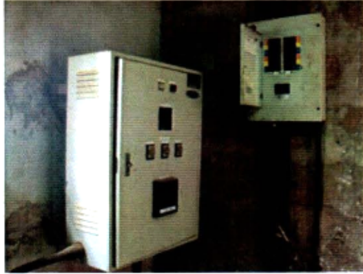
Plate XXXVII: Program-Controller and Main Switch.
