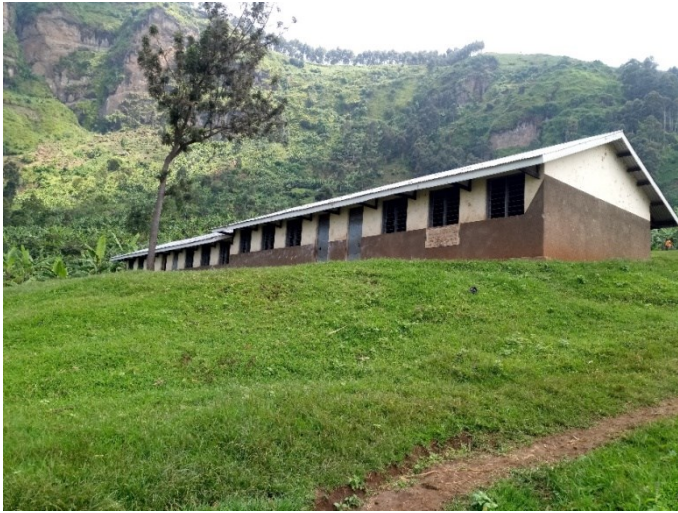
4-classroom block – front
