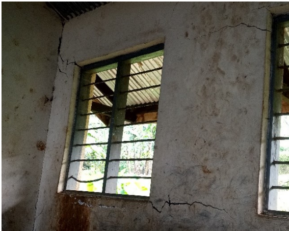
Other cracks on wall and aprons - Effect of moisture due to poor drainage around the structures
