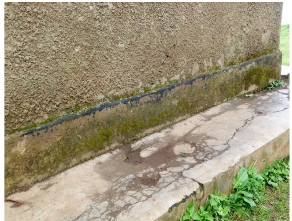
Other cracks on wall and aprons - Effect of moisture due to poor drainage around the structures
