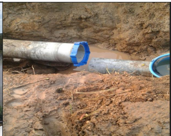
Repair works on PVC pipes
