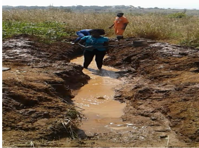
Pipe exposure to facilitate repair
