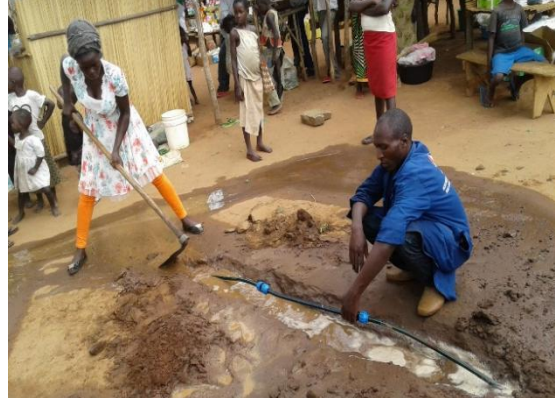
Repair works on burst
