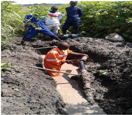
Repair works on Distribution line
