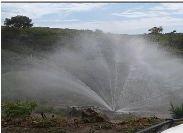
Burst on the mains
