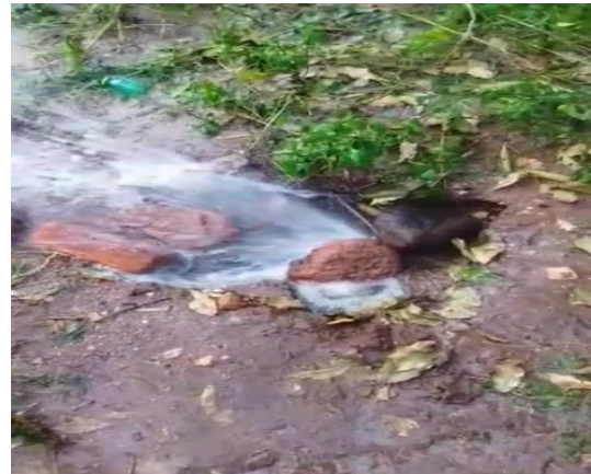
Losses from a pipe that has been cut
