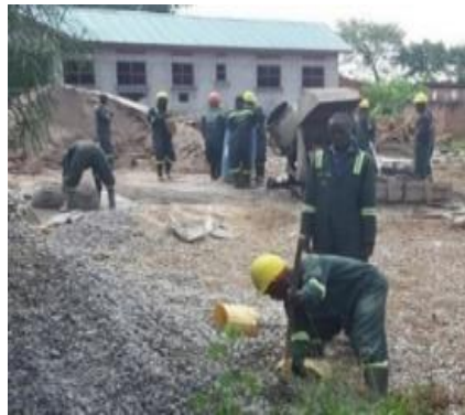
( c ) Material handling on a construction site
