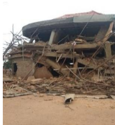
(e) Collapsed building in Kampala
