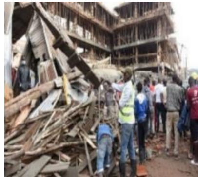
(f) Collapsed building in Jinja city
