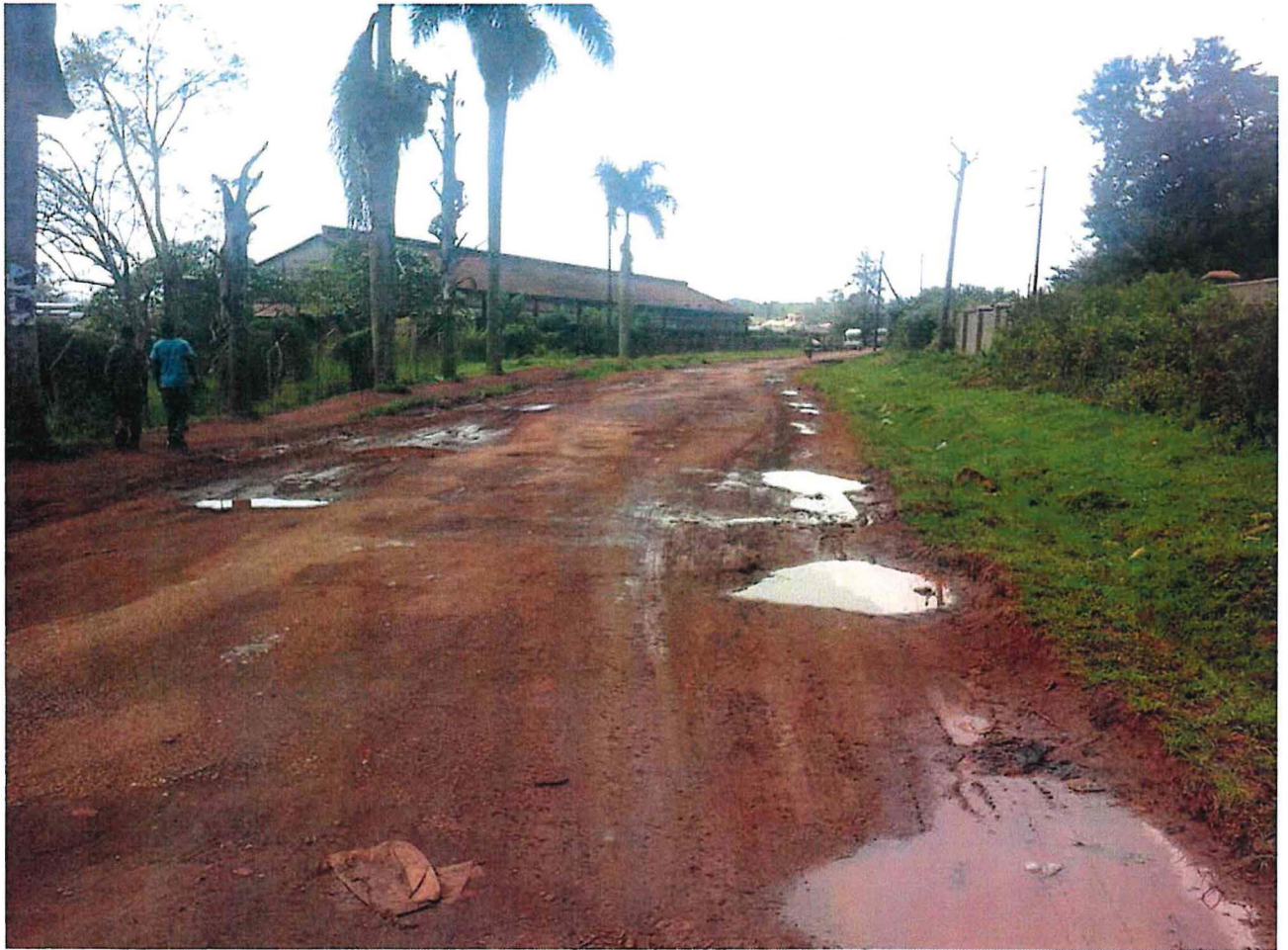
Photo 5: Potholes and Bushes along roads along Yusuf-Lule Road
