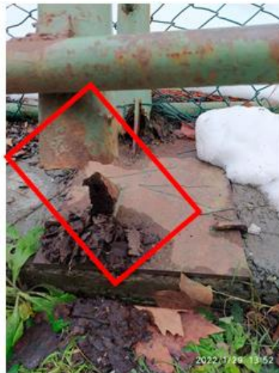
Figure 1-1: Corrosion damage to structural members that ended up collapsing (Fırat Alemdar et al., 2023)
