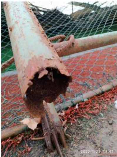
Figure 1-1: Corrosion damage to structural members that ended up collapsing (Fırat Alemdar et al., 2023)
