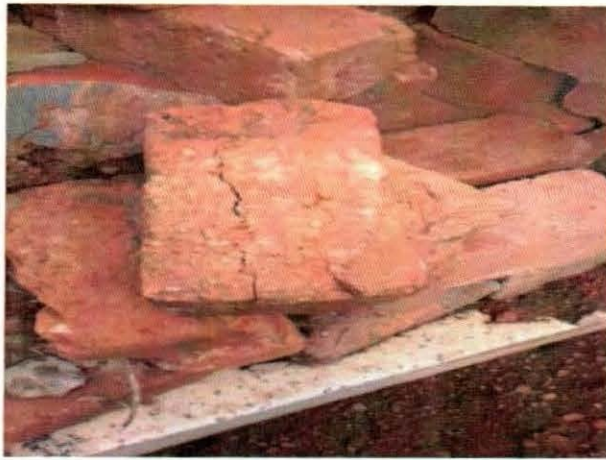
Figure 1.2 : Cracks and breakages of burnt clay brick
