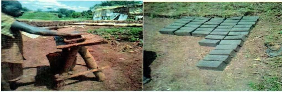
Figure 4.8: Artisan method of brick molding
