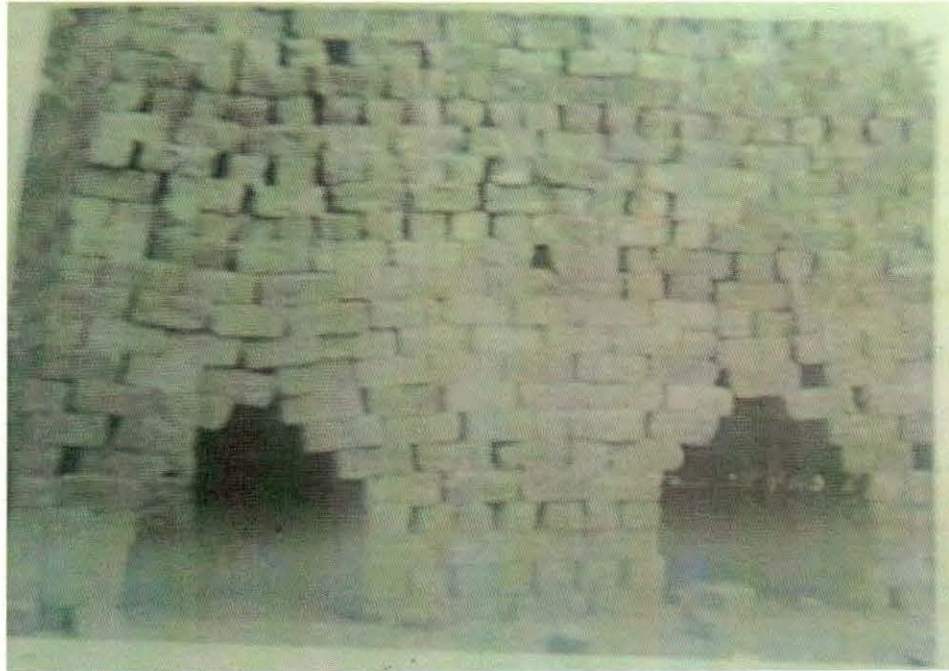
Figure 4.9: Field Kiln for burning of bricks and cooling
