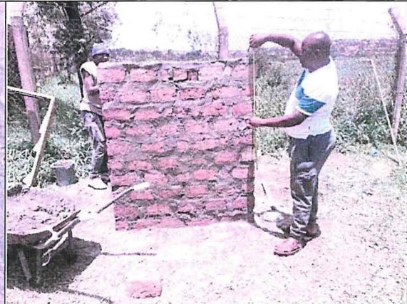
Measuring the specified height of the setup
