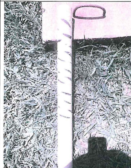
Percolate pipe drilled with holes.
