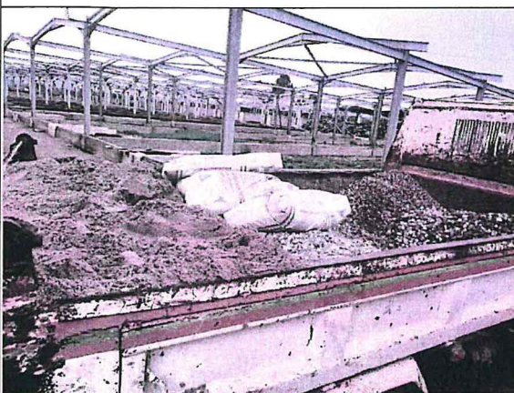
Materials for the set-up of the site
