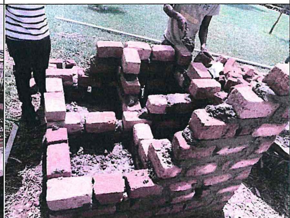
Experimental set-up construction
