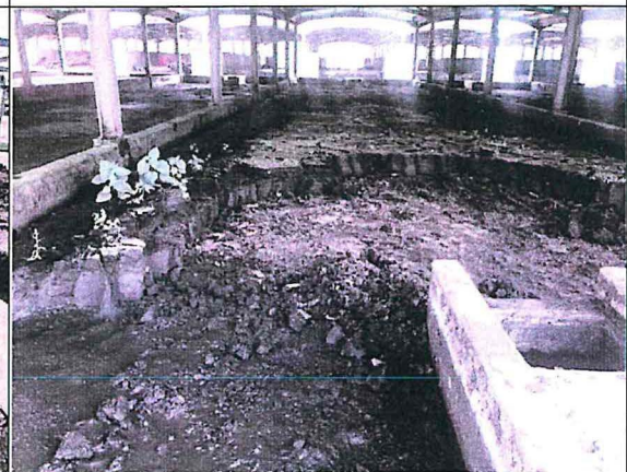
Sludge cakes being removed
