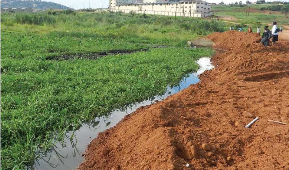
Figure 2: In-Filling of Murram in Nakivubo Wetland
