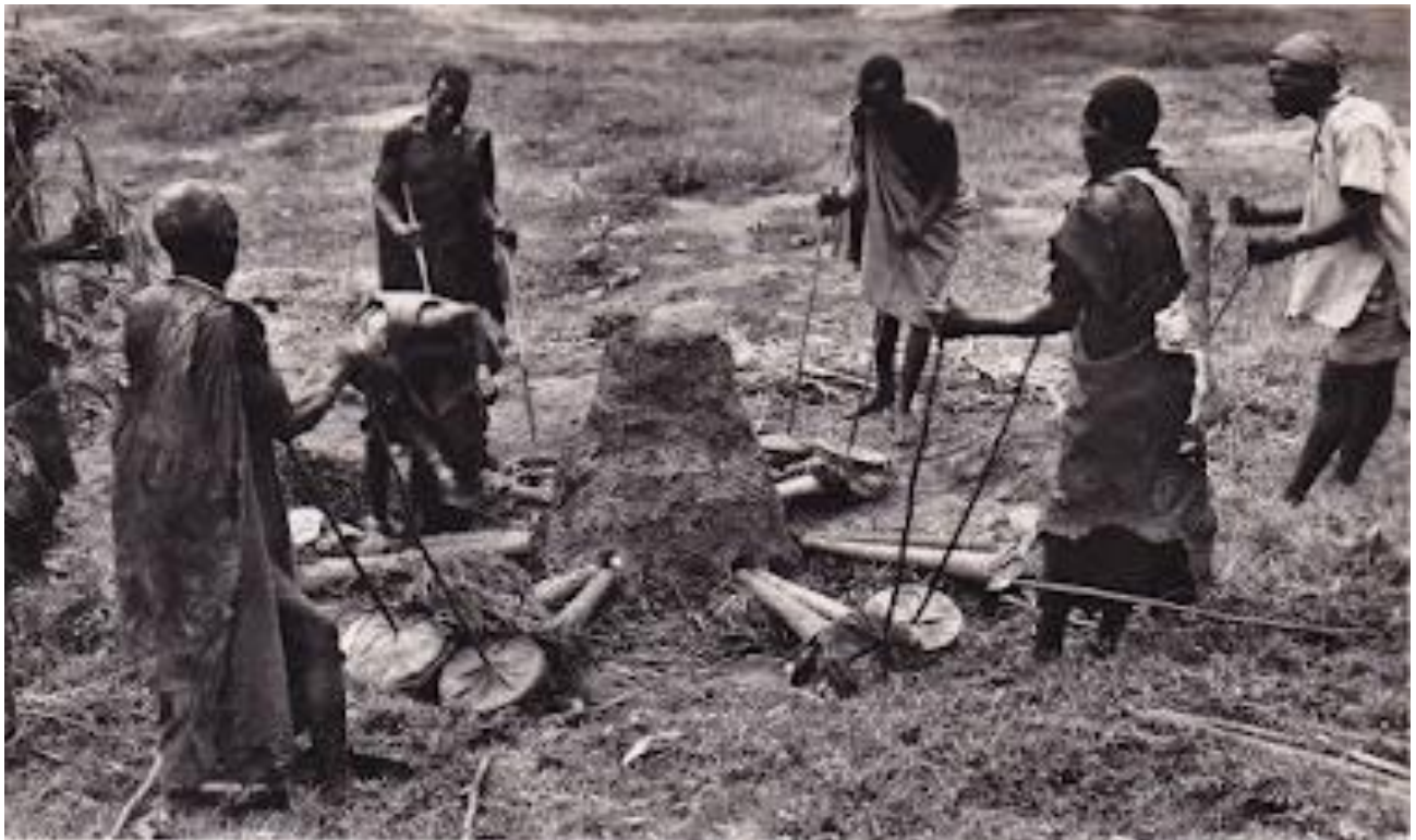
Figure 21: Native Iron Smelter of Kigezi, South-western Uganda
