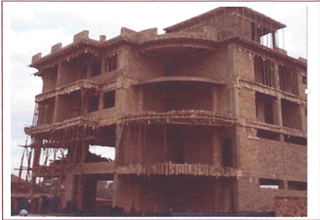
Figure 0-2: Reinforced Concrete framed structure with burnt clay bricks infills.
