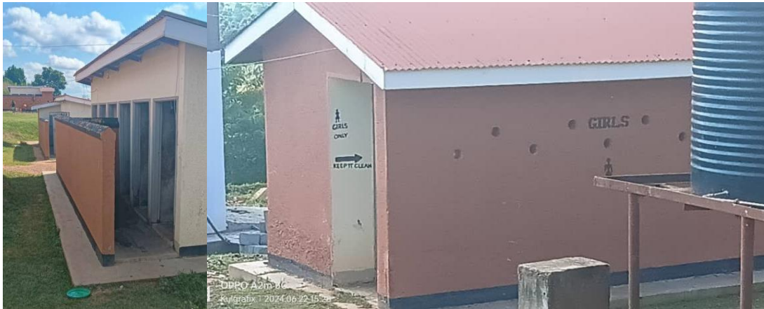
Figure 12: Toilet facilities for the boys (l) and girls (r) in the school.
