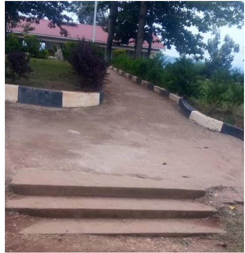
Figure 2: Pathway with steps and a ramp on the right-hand side.
