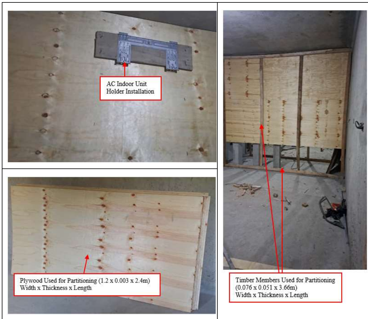
Figure 3. 4: Experiment room setup with timber, plywood and concrete floor/ceiling
