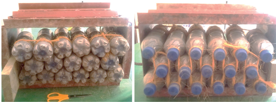
Figure 6. Tying PBB masonry units.
