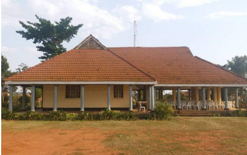
Figure 4: Former District Administrative Building in Maluku Sub County, Mbale
