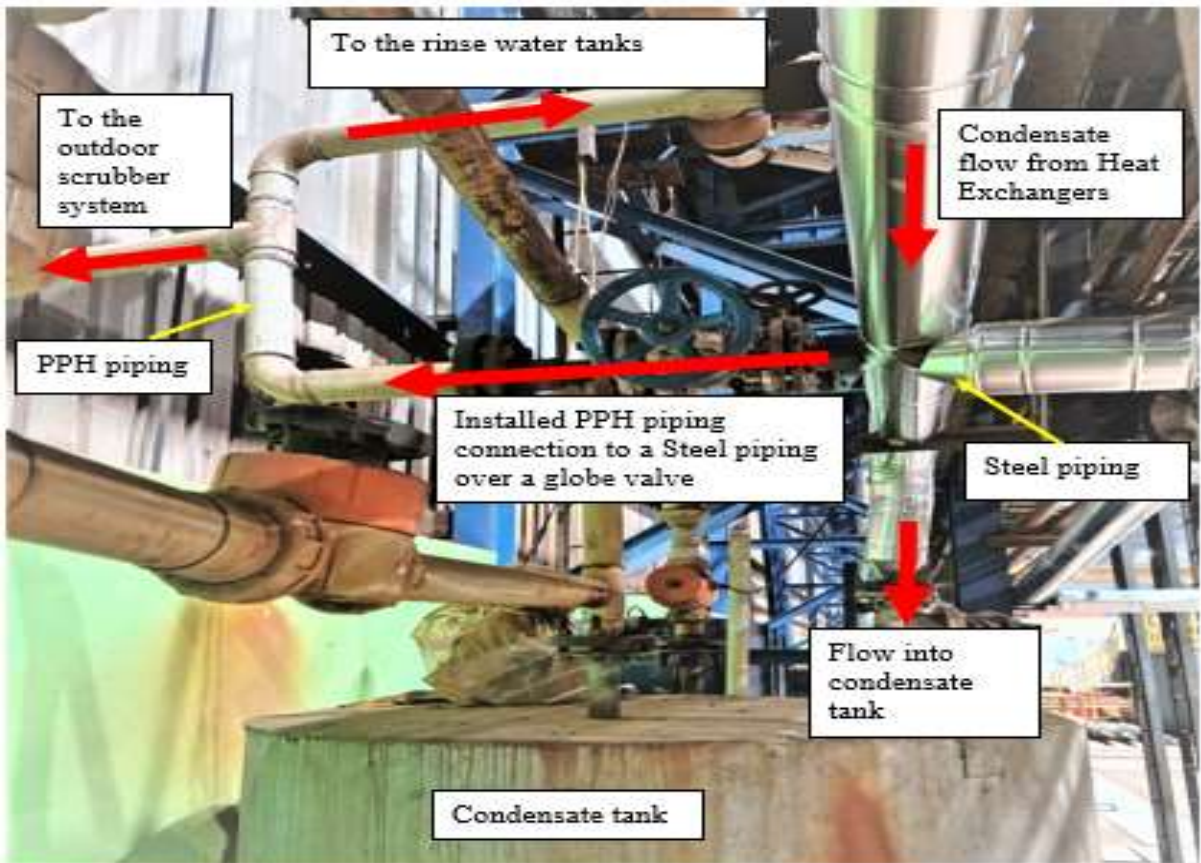
Figure 3-2. A Portion of a steel piping replaced with PPH piping
