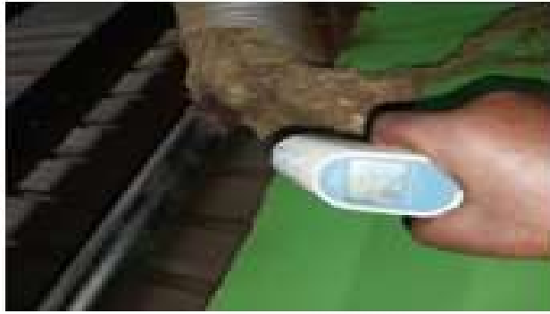
(a) Temperature of uninsulated steel elbow
