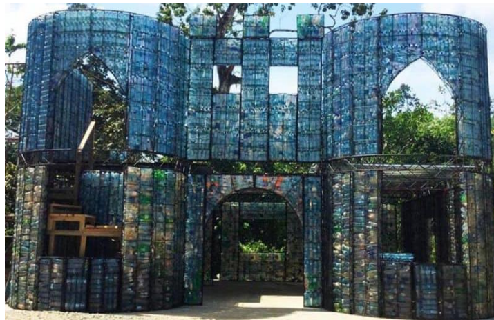
Figure 2-1: Construction of the plastic bottle village, located on the island of Bocas del Toro in Panama.
