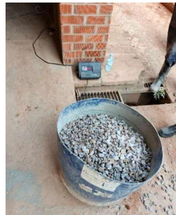
d. Weighing of coarse aggregates before mixing
