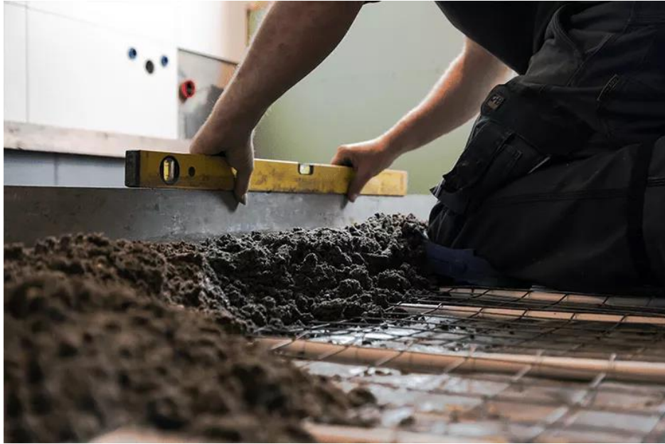
Figure 2- 7: Leca lightweight aggregate concrete as a fill material
