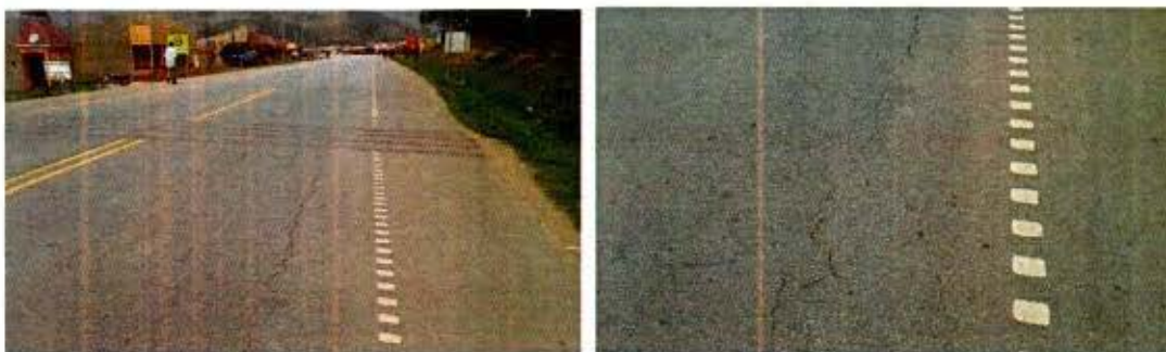
Figure 2.7: Asphalt concrete surfacing along Mbarara - Kabale section
