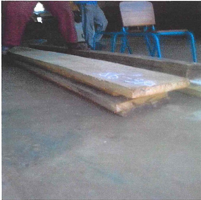
Fig.16 showing the new boards
