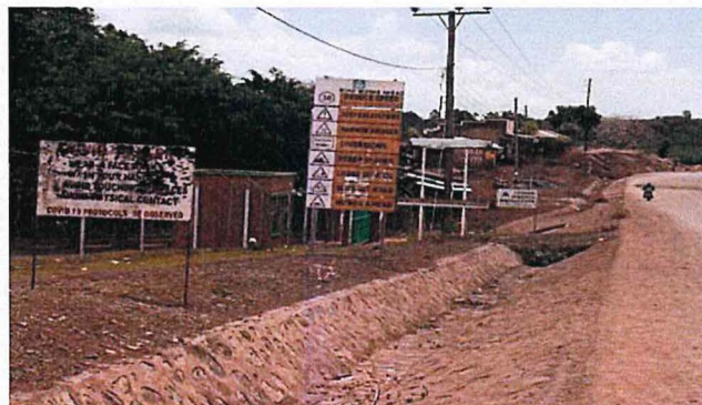
Plate 19. The newly rehabilitated highway without FGM signage
