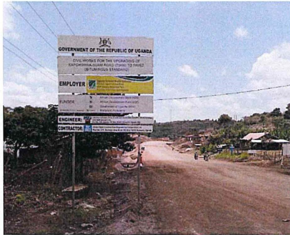
Plate 20. Signage displaying Civil works for the upgrading of Kapchorwa Suam road 73km to paved Bituminous standard.
