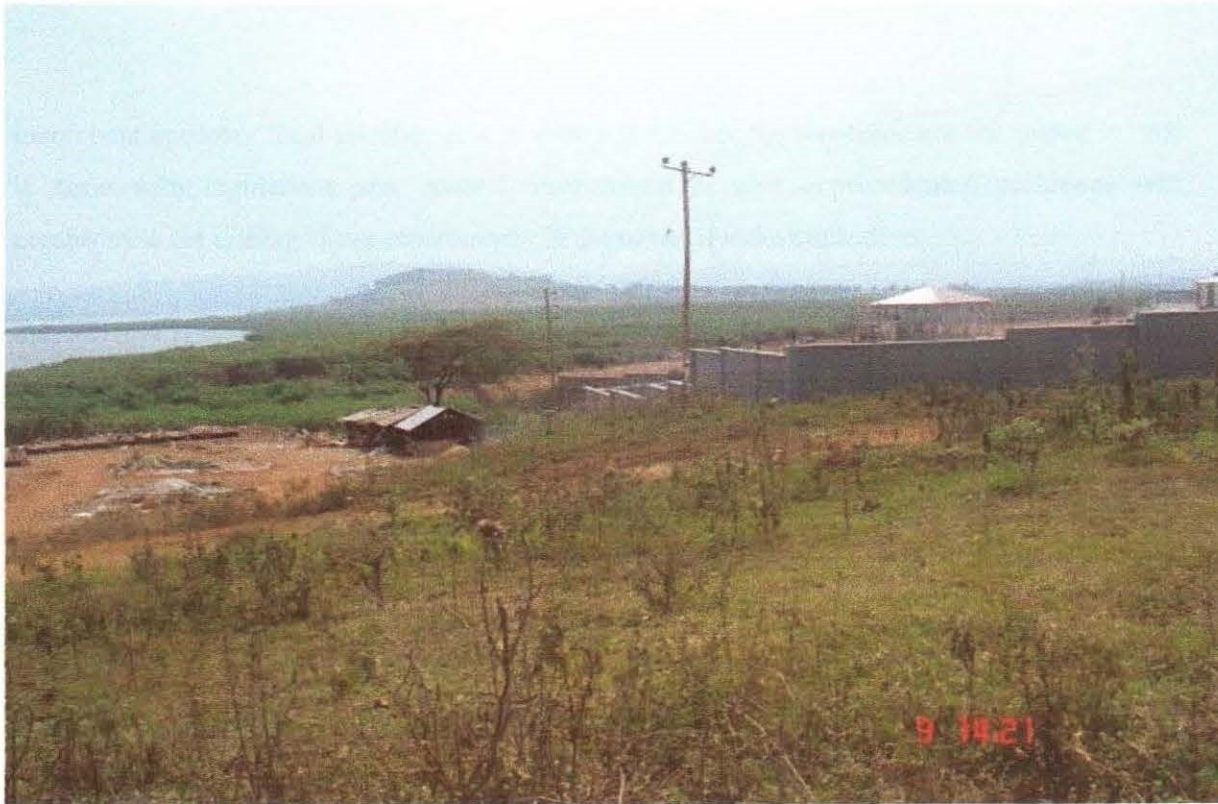
Fig 4.20 : Industrial activity encroaching on a wetland
