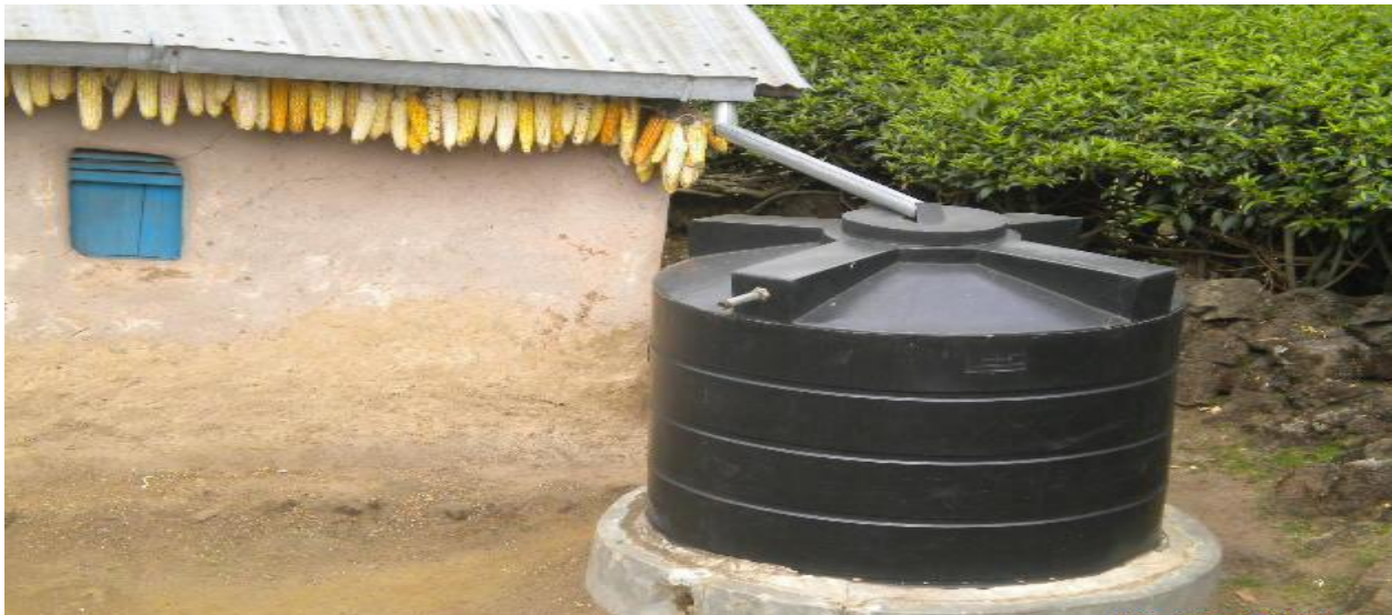
Figure 4.6: One of the rain harvesting tanks provided by Compassion international
