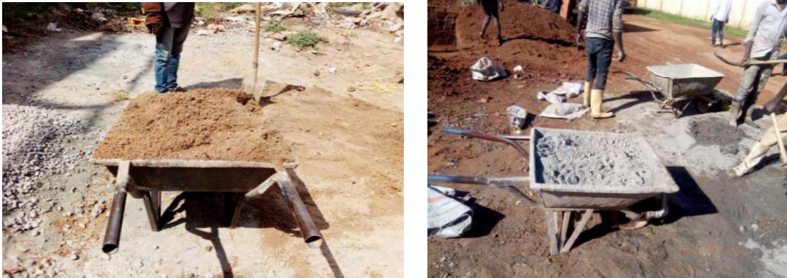
Figure 4. 1: Wheel barrow full of sand and wheelbarrow of cement (50 kg bag cement)
