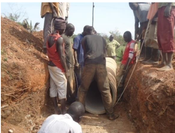
Installation of 600mm diameter reinforced concrete culverts taking place
