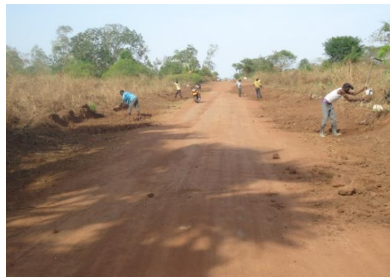
Manual excavation to level to form a levelled road bed
