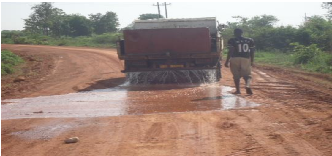
Watering of road section
