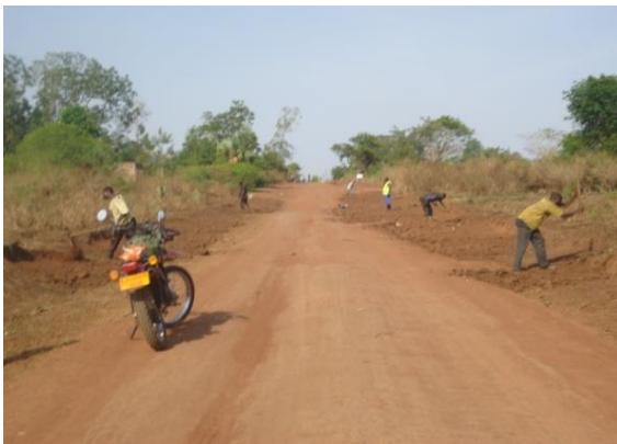
Manual excavation to level to form a levelled road bed
