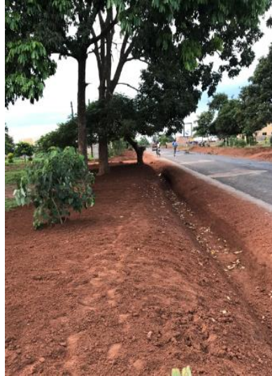
Side drain improved manually
