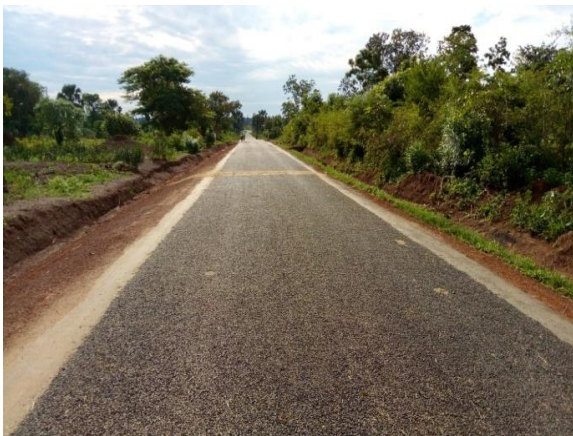
A completed SSD section
