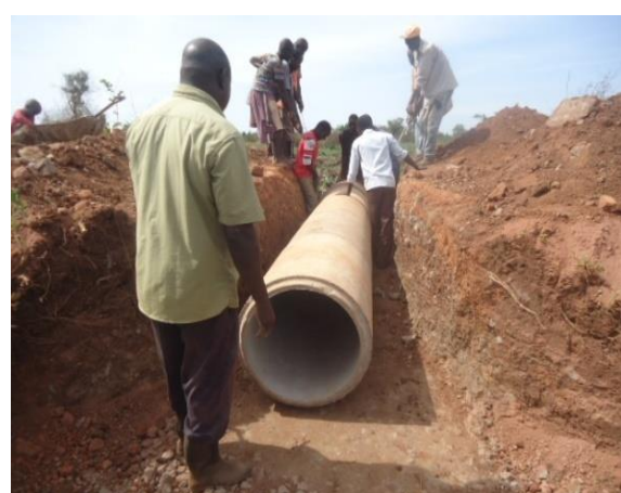
Installation of 600mm diameter reinforced concrete culverts taking place
