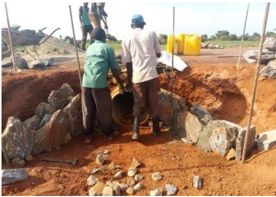
Construction of head and wingwalls in progress
