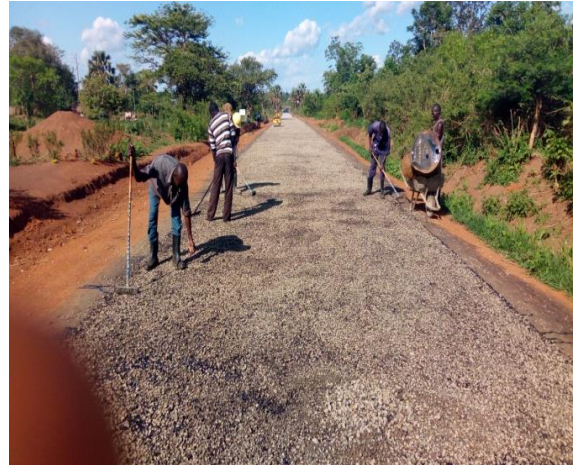
10-14mm stone chippings laid on K160
