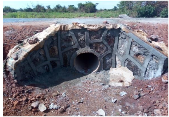
Completed head and wingwalls
