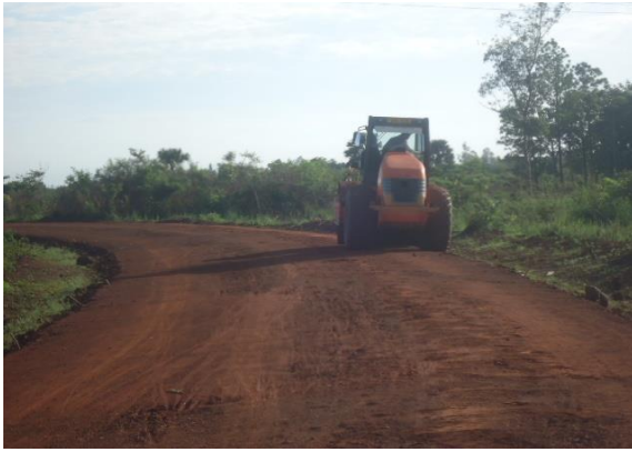
Compaction taking place
