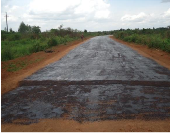
MC30 primer to clean the road surface
