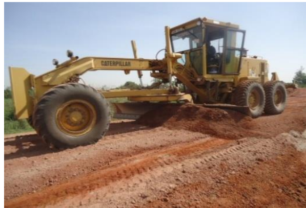
Spreading stabilized gravel using a Grader
