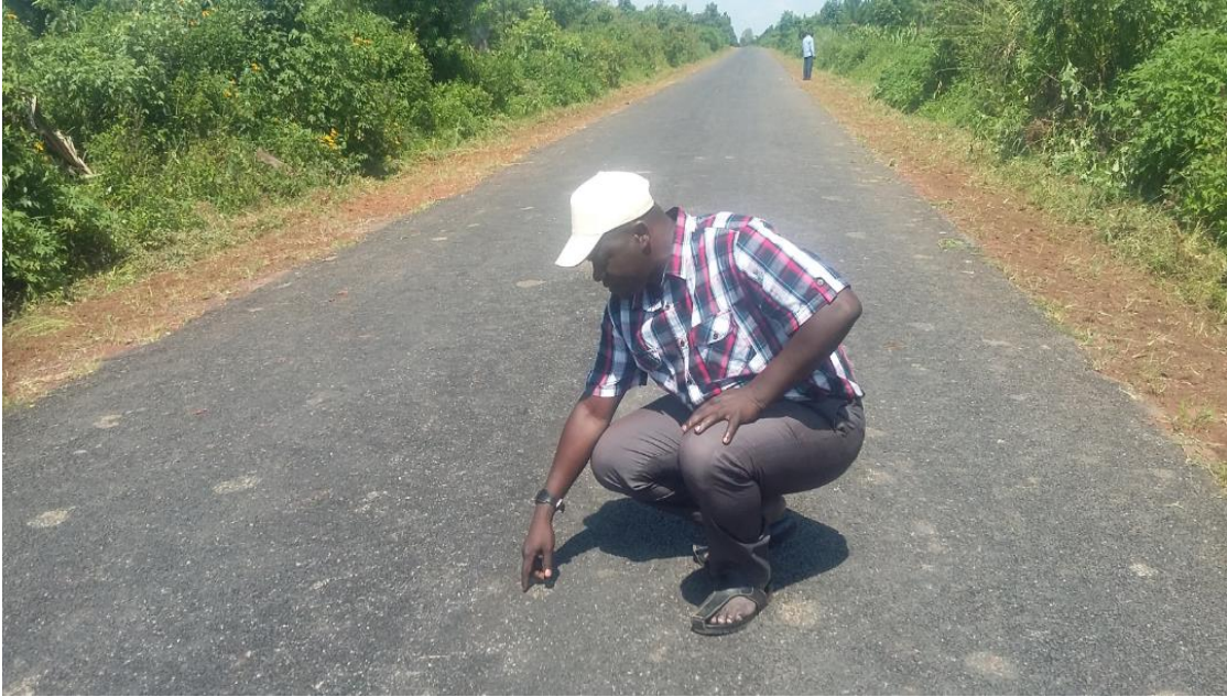
A completed section of SSD in Kole district using mix method of grader and labour
