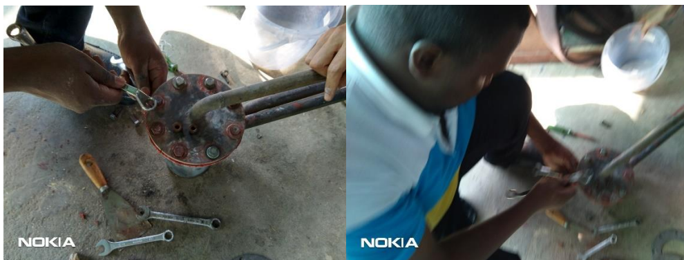
Nut fastening of the reactor containing the biomass.
