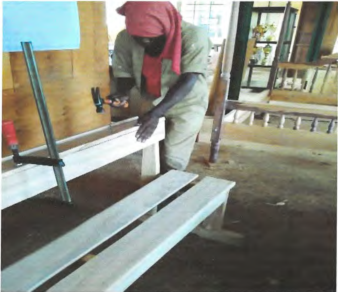
Fig.28: Two pieces of timber due for nailing held together with an F. clamp for firmness. Learner did not need a helper (Source: Primary Data 2018 )
