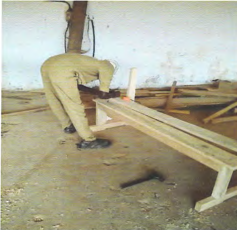
Fig.24: Learner Framing up a church pew, a tape measure to ensure correct measurements as per from the working plan (Source: Primary Data 2018)
