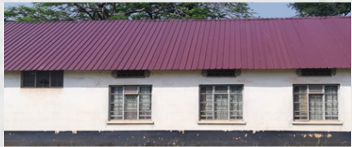
Completed Roofing of main stores where asbestos iron sheets were removed
