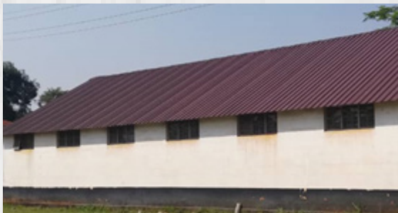
Completed Roofing of main stores where asbestos iron sheets were removed
