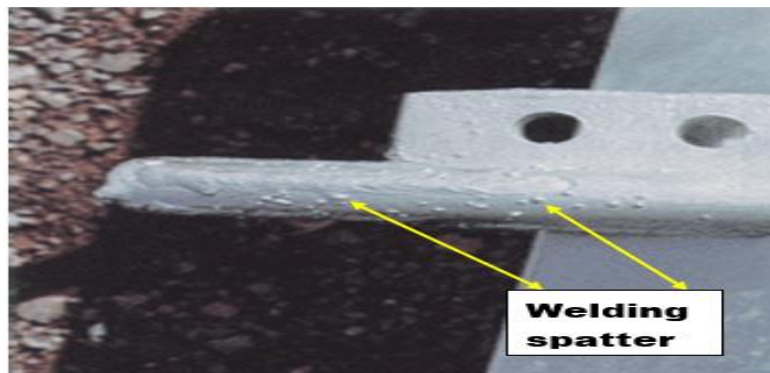
Figure 2-16 : Welding Spatter (AGA, 2016)
