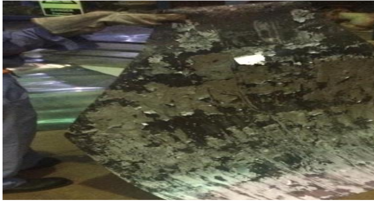
Figure 4-4 : Rejected sheet - black spots (on site pictures)
