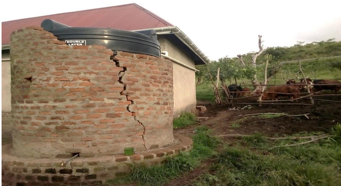
Plate 4.3: Photograph showing rainwater harvesting plastic tank in Kibimbiri village, Bweramule Sub County
