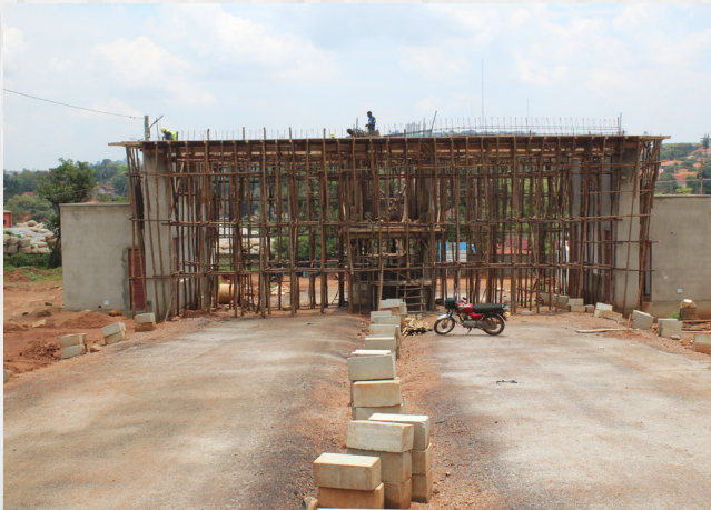
On going construction of the West end main gate
