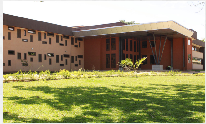
Technical Teacher Facility with lecture rooms
