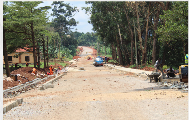
On going construction on Fisher road
