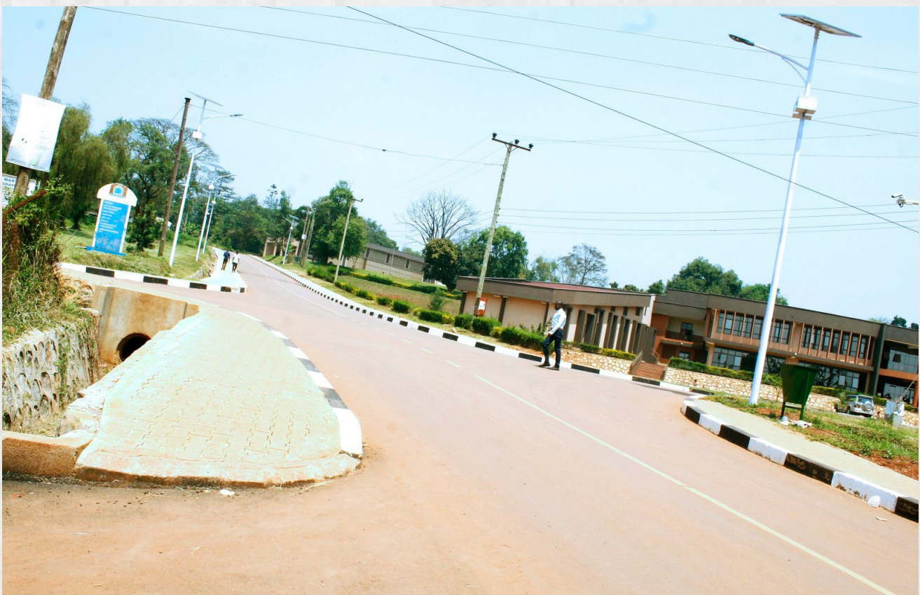
The new Harlow Road
