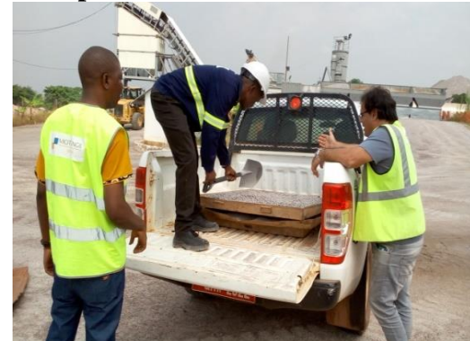
Figure 3.5: Loading hot aggregate on pickup
