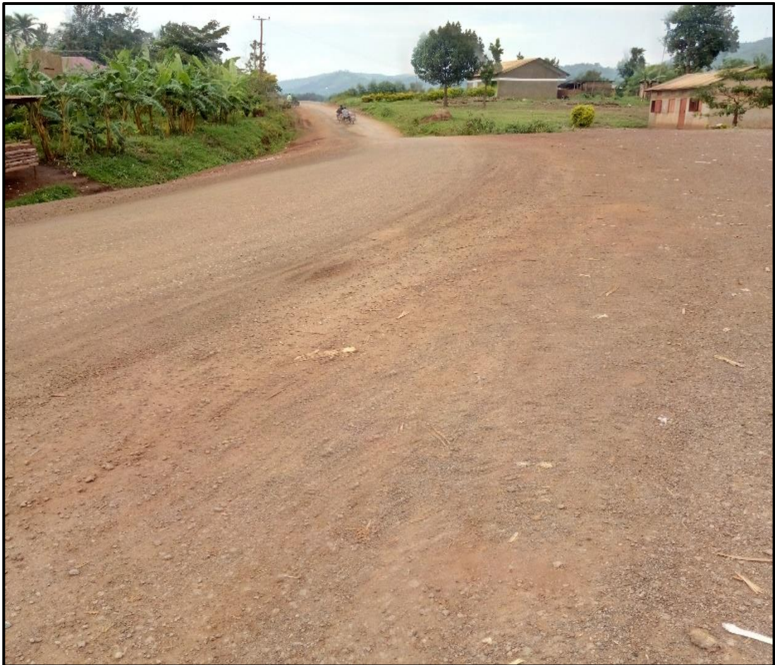
Figure 4.8 Section of road where the contractor was blocked from work at chainage 1+970-2+200
