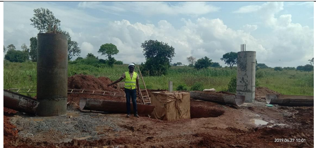
Support piles already cast on site
