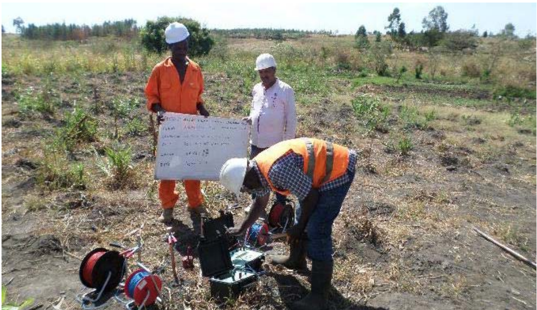
Figure 3.5: Soil resistivity measurement in the field
