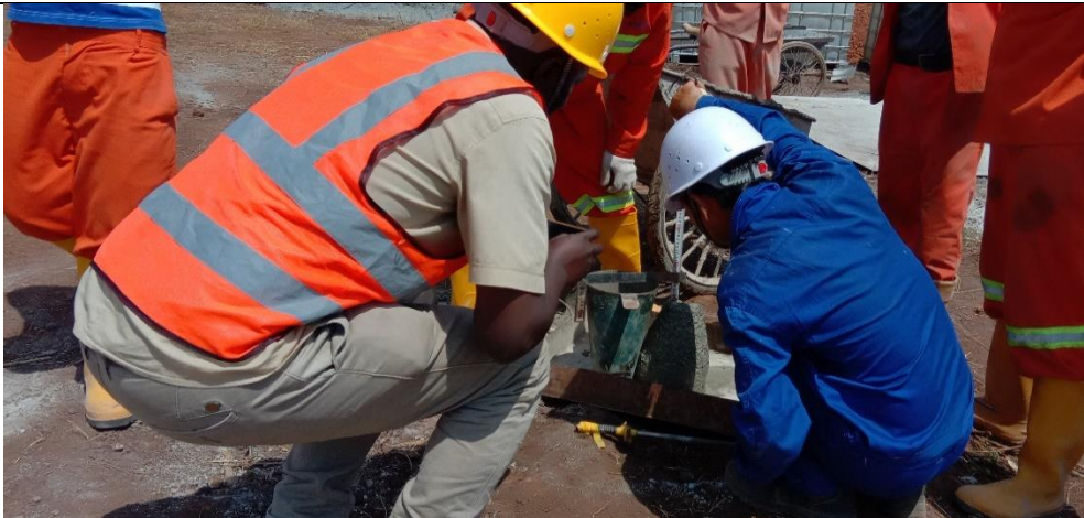
Site QA/QC checks for slump
