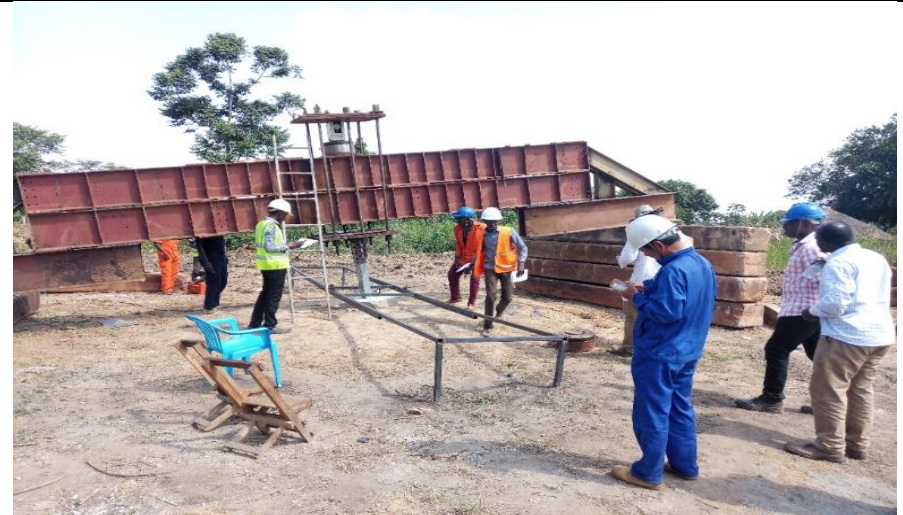
Commencement of uplift Test at KL 30
