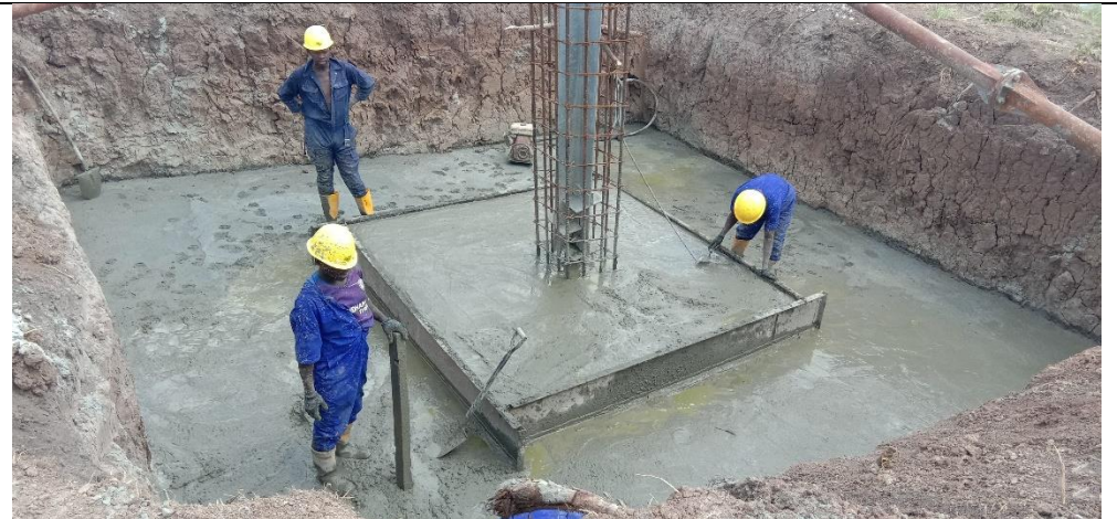
Concrete Casting for the Step-Pad foundation section
