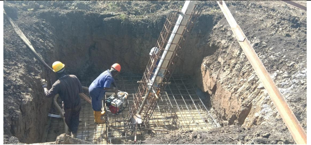
De-watering of the Foundation pit
