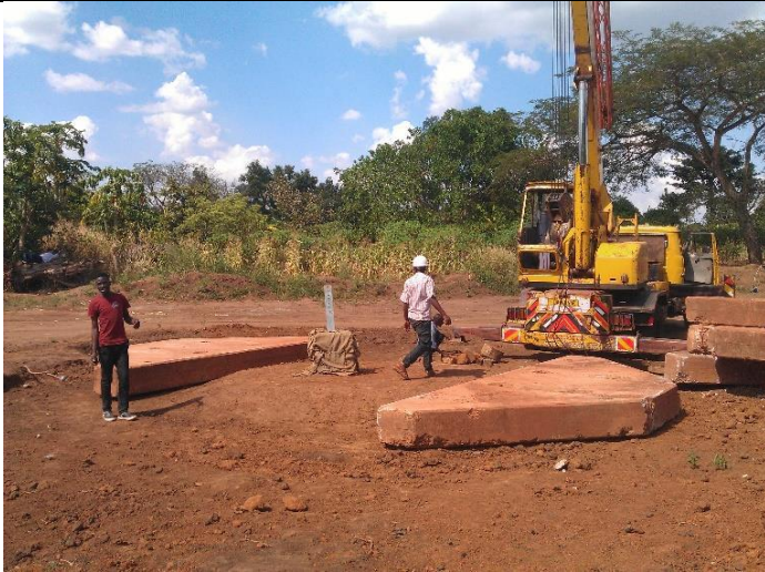
Static Uplift/Tension Load Testing setup
