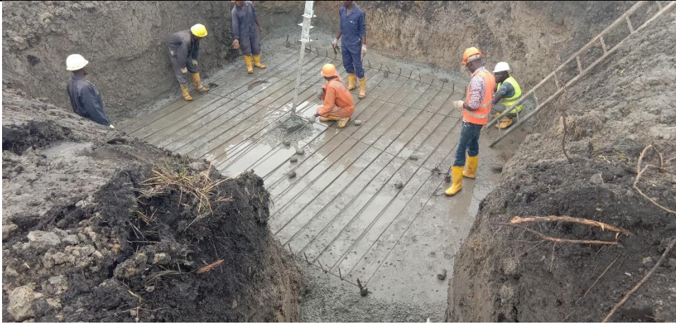
Rebar assembly after completion of foundation excavation
