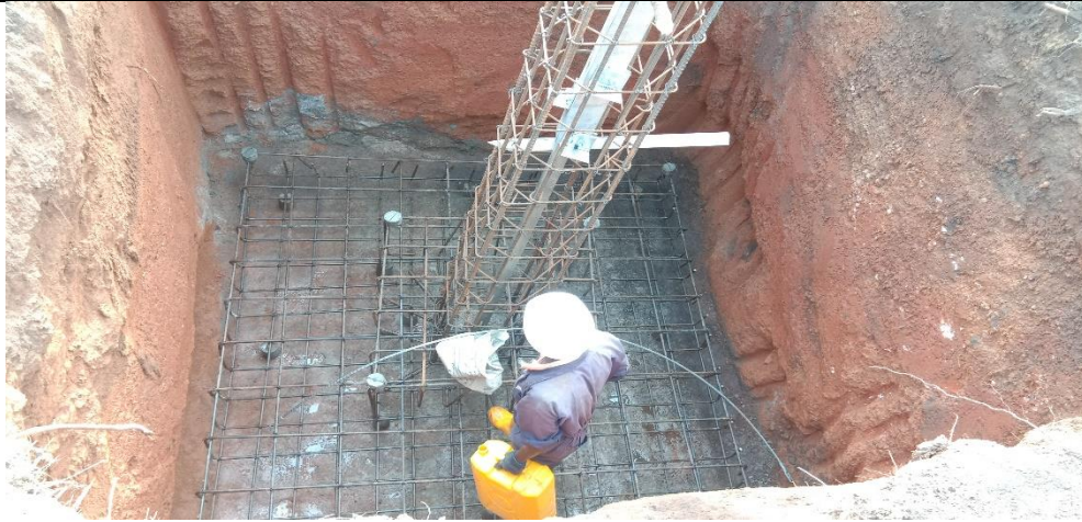
Rebar assembly after completion of excavation works
