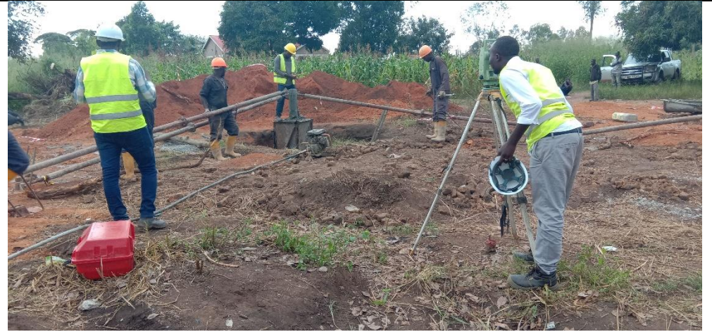
Level checking on site by the Researcher
