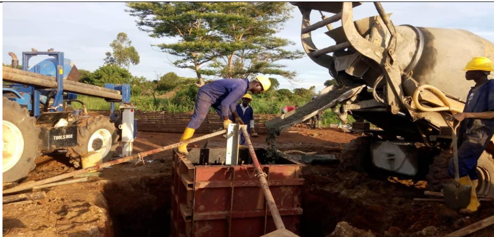
Pile cap concrete casting
