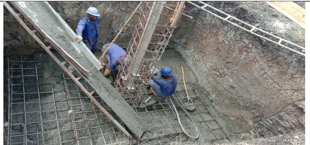
Preparations for pad and column/chimney concrete casting
