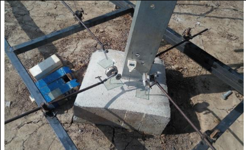
Ground situation during the test at KL 30
