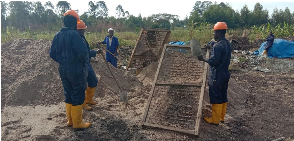
Sand Sieving works ahead of concrete casting
