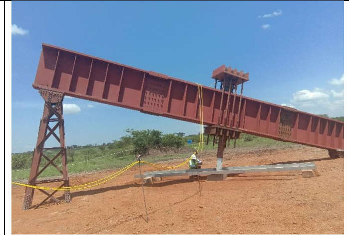
Completion Photo - Static Axial Uplift Load Test
