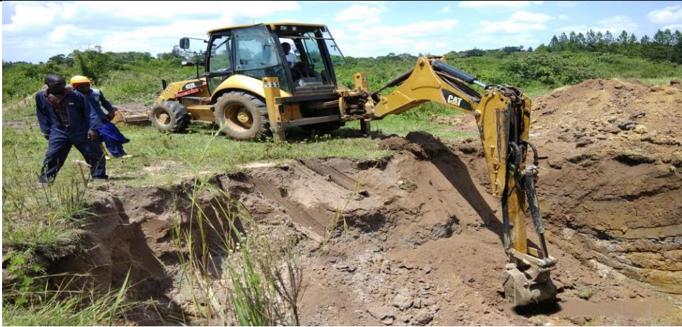
Excavation works ongoing
