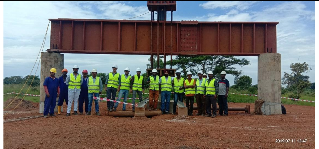
Static Axial Tension/Uplift Load Test
