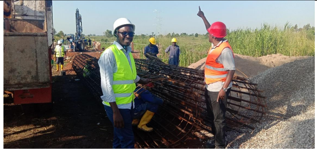
Rebar tying and assembly inspections
