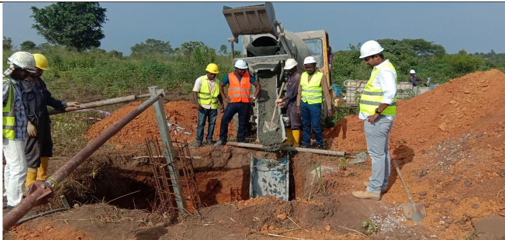
Concrete casting of Pad and Chimney foundation
