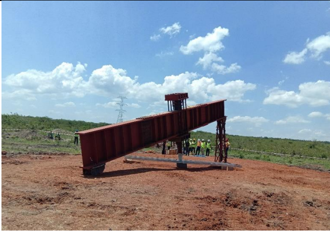
Static Axial Tension/Uplift Load Test
