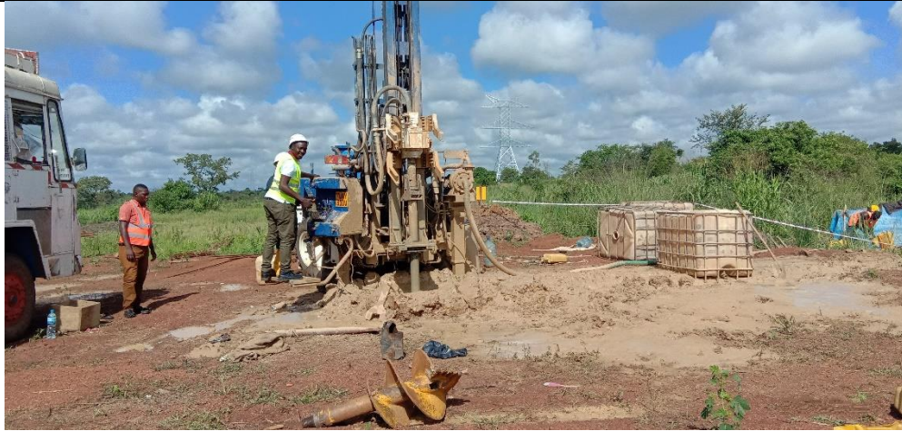
Pile (900 mm diameter) boring excavation works
