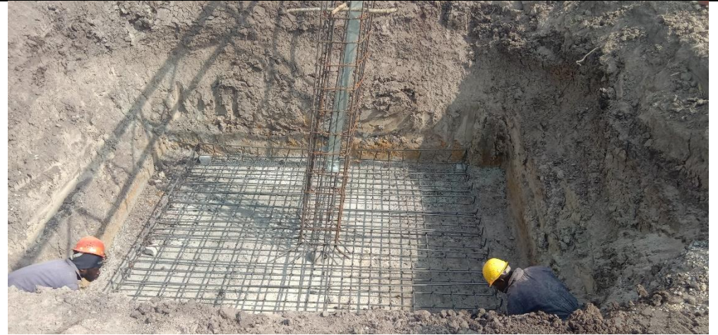
Rebar assembly and pit side cutting
