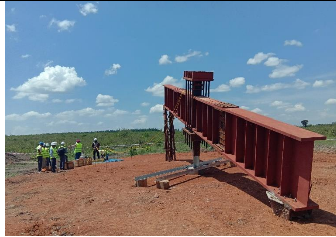
Static Axial Tension/Uplift Load Test
