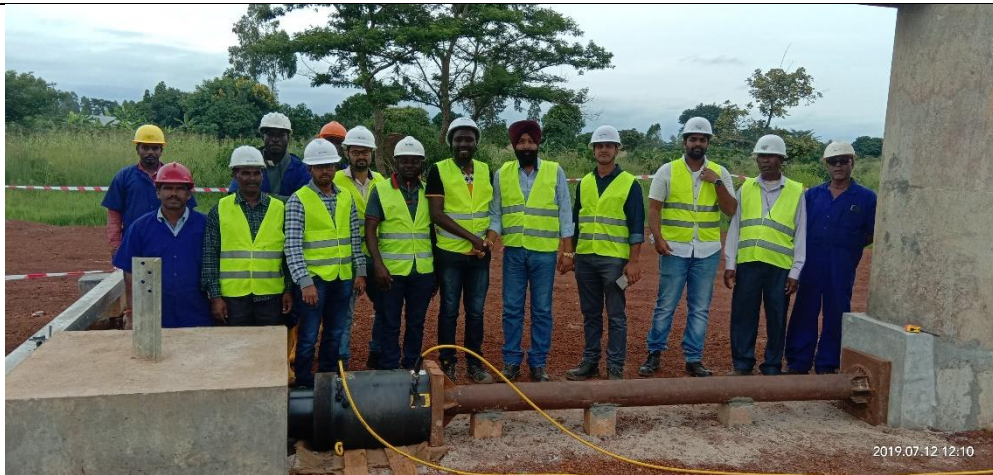
Lateral Load Foundation Test
