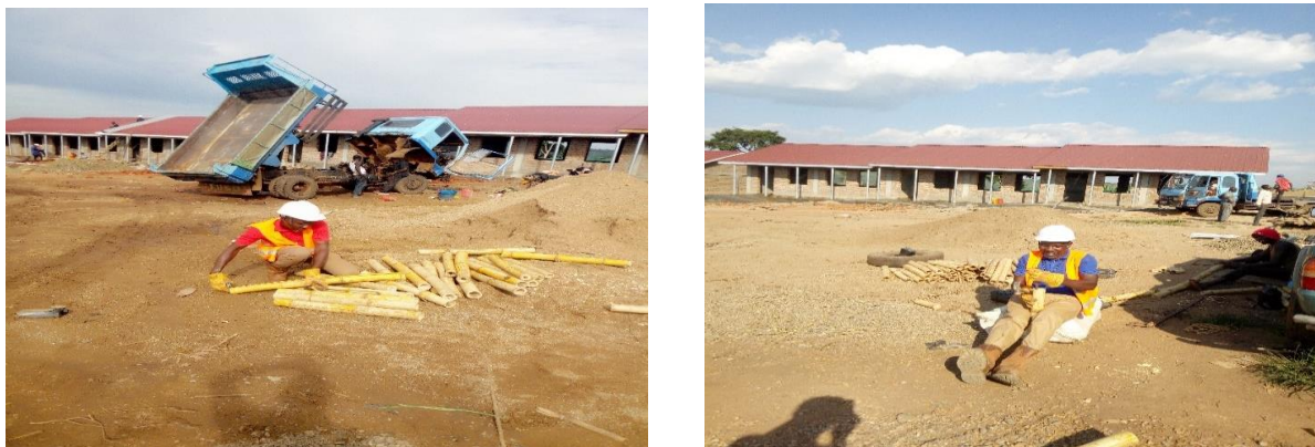
Figure 3.4: Cutting the bamboo samples to the desired lengths and Right: Opening the bamboo Culms using an improvised chisel and hammer.
