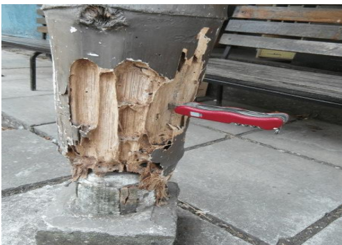
Figure 2.9: Bamboo attack by termites
