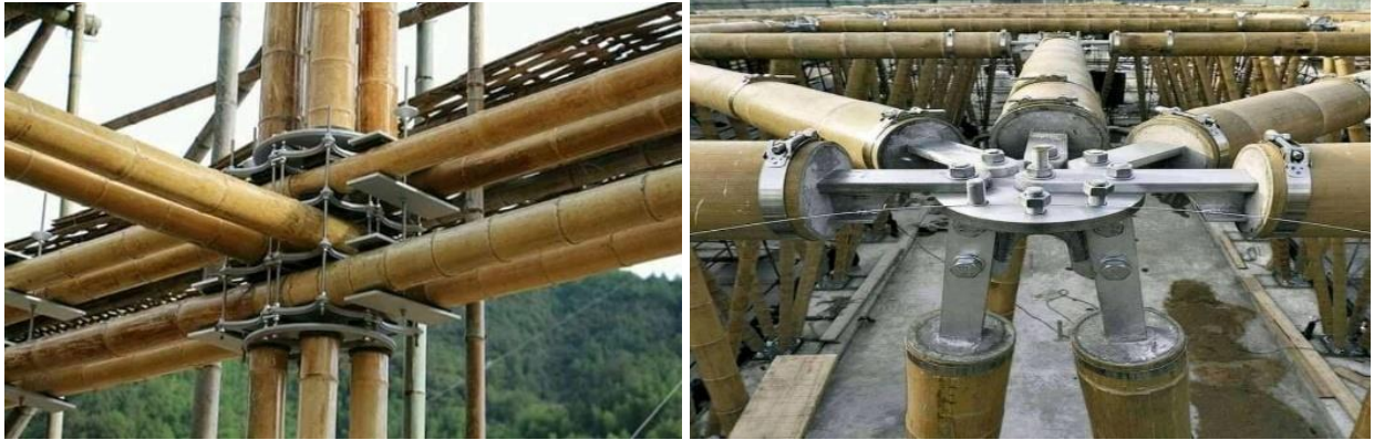
Figure 2.2: Jointing and connections of bamboo culms.
