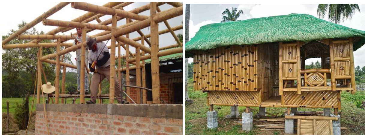
Figure 1.2: Plain bamboo used as columns and trusses and as decorative walling material.
