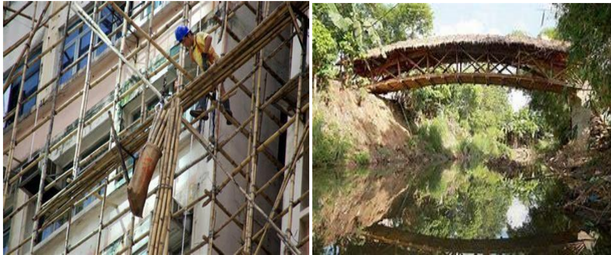
Figure 1.1: Structural use of bamboo as scaffolds (left) and as a bridge (right)
