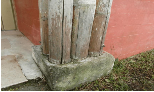
Figure 2.10: Boron-treated bamboo culms splitting and bleaching when exposed to sun and rain.
