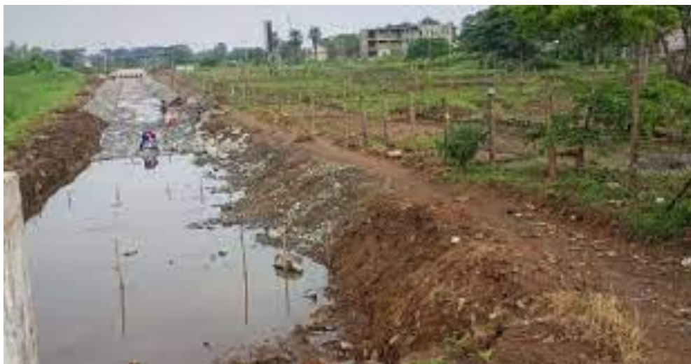
Figure 4. 3: Poor land use causing poor drainage
