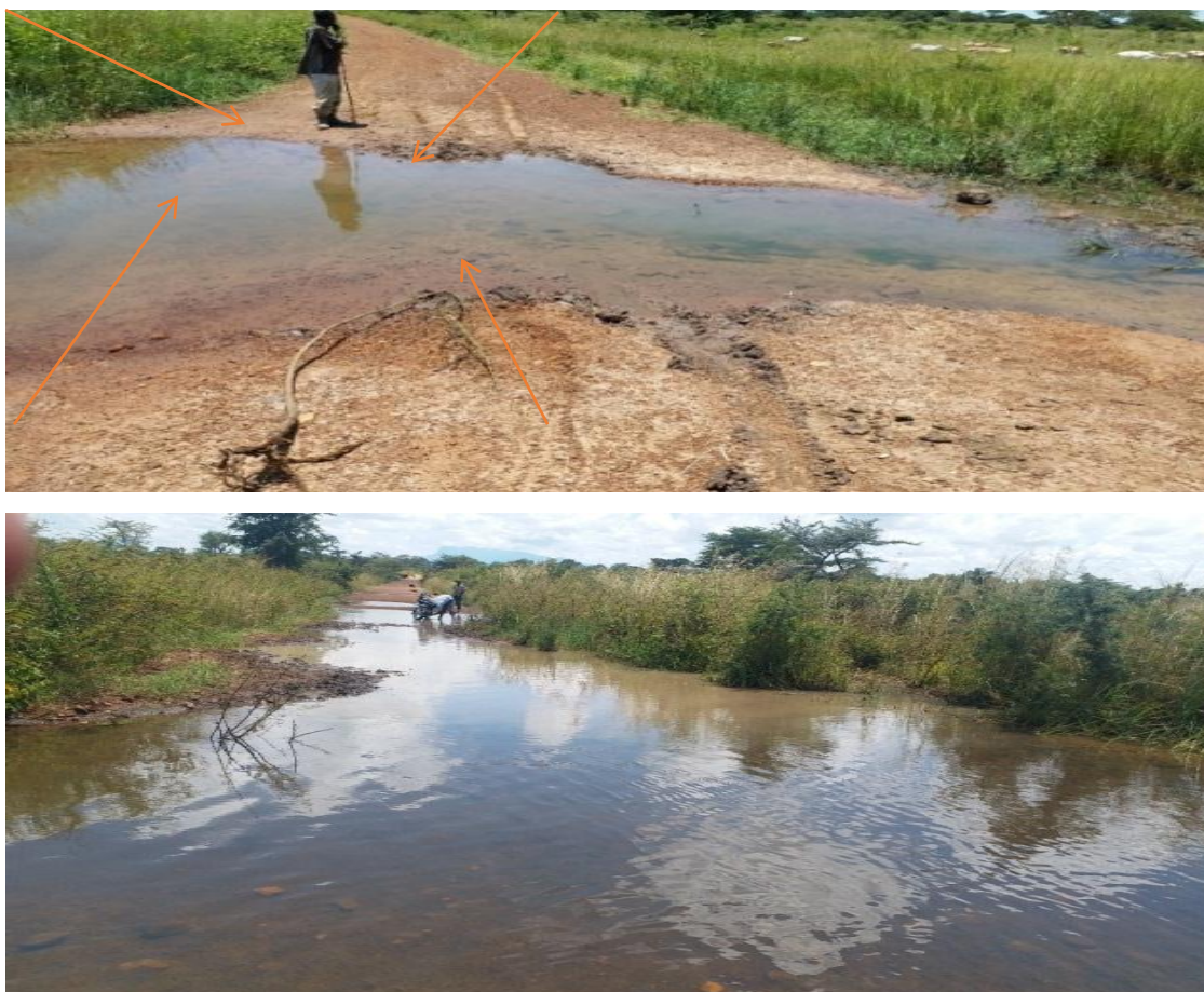
Figure 4. 4: Poor drainage along Usuk-Ongongoja road
